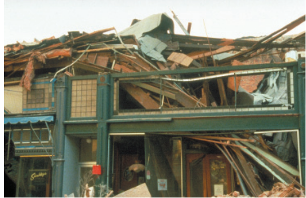
■ Figure 5. Destruction of a historic building.
