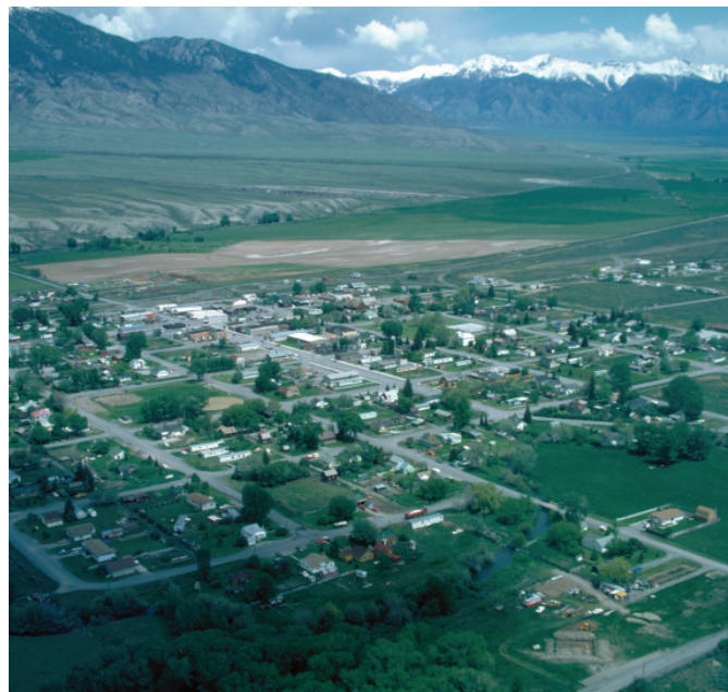
■ Figure 17. Aerial view of heavily damaged Mackay, Idaho. The unreinforced masonry buildings on the main commercial street of the small town were badly damaged in the 1983 Borah Peak, Idaho earthquake. —NISEE, U.C. Berkeley
