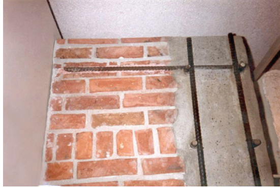
■ Figure 31. California Capitol Retrofit.
