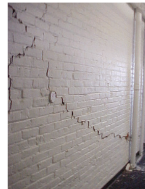
■ Figure 19. URM building damage, 2001 Nisqually, Washington earthquake.
