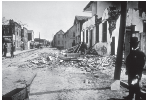
■ Figure 13. Debris resulting from the 1886 Charleston, South Carolina earthquake. —NISEE, U.C. Berkeley
