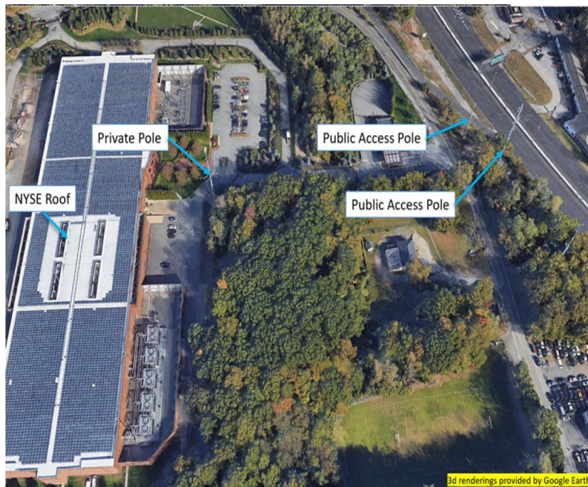
Figure 4: Mahwah Data Center 1
