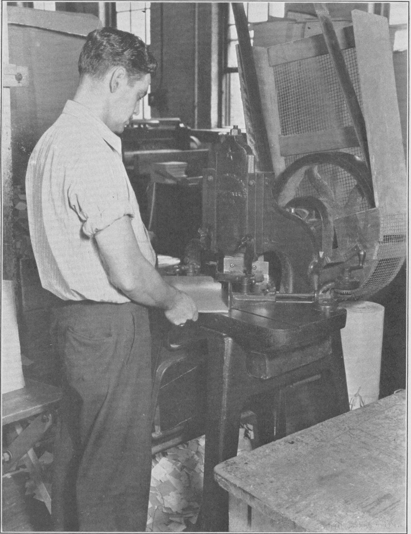
PLATE 6.—CUTTING OUT CORNERS OF BOARD BLANKS ON A SINGLE-CORNER CUTTING MACHINE.
