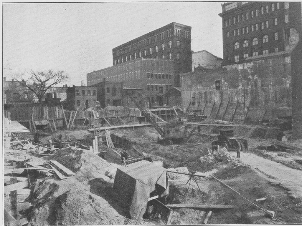
Excavation and test boring work in progress on the new addition to the Government Printing Office
