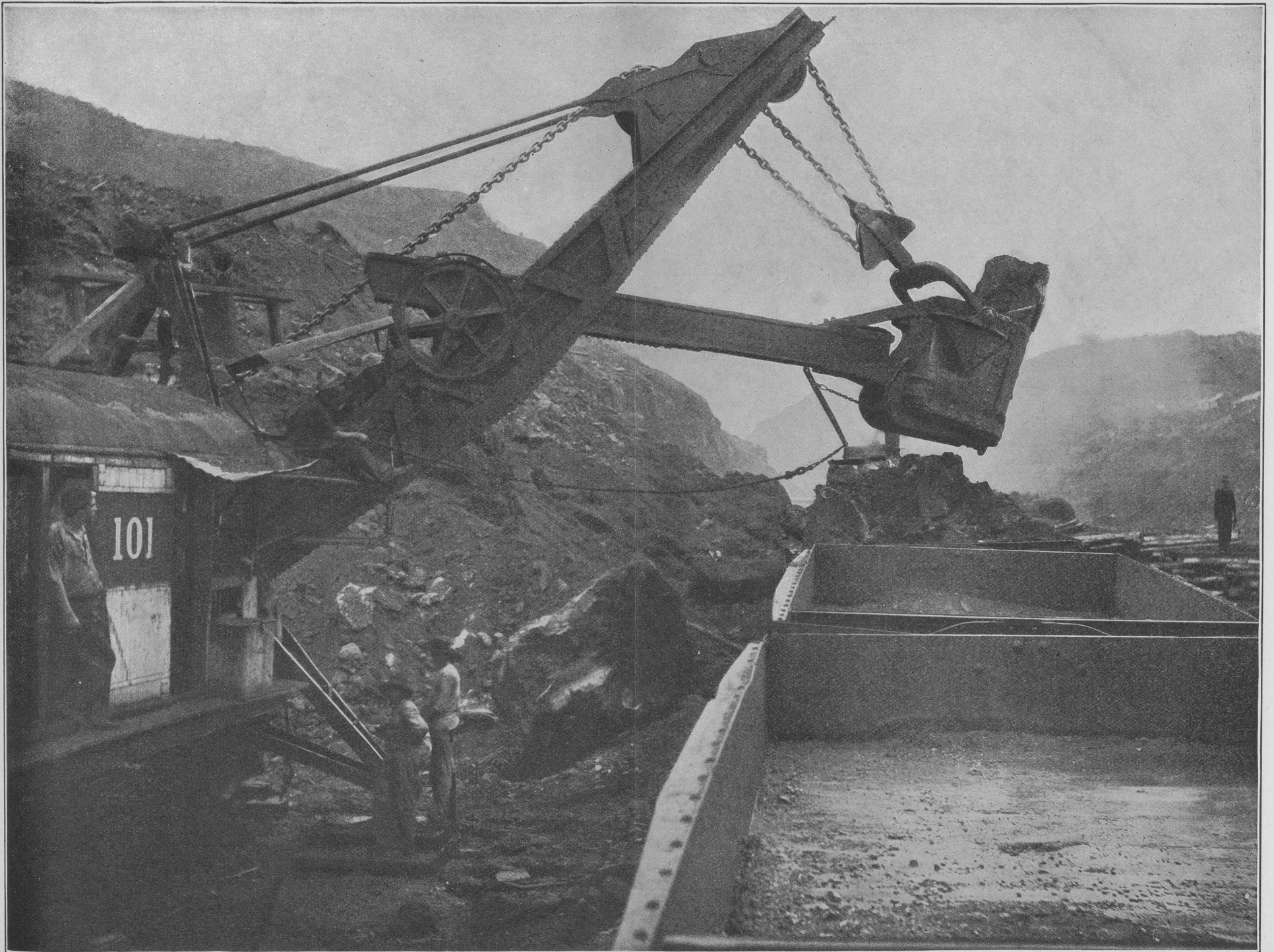
STEAM SHOVEL AT WORK IN CULEBRA CUT, WITH LARGE ROCK IN MOUTH OF SHOVEL.
