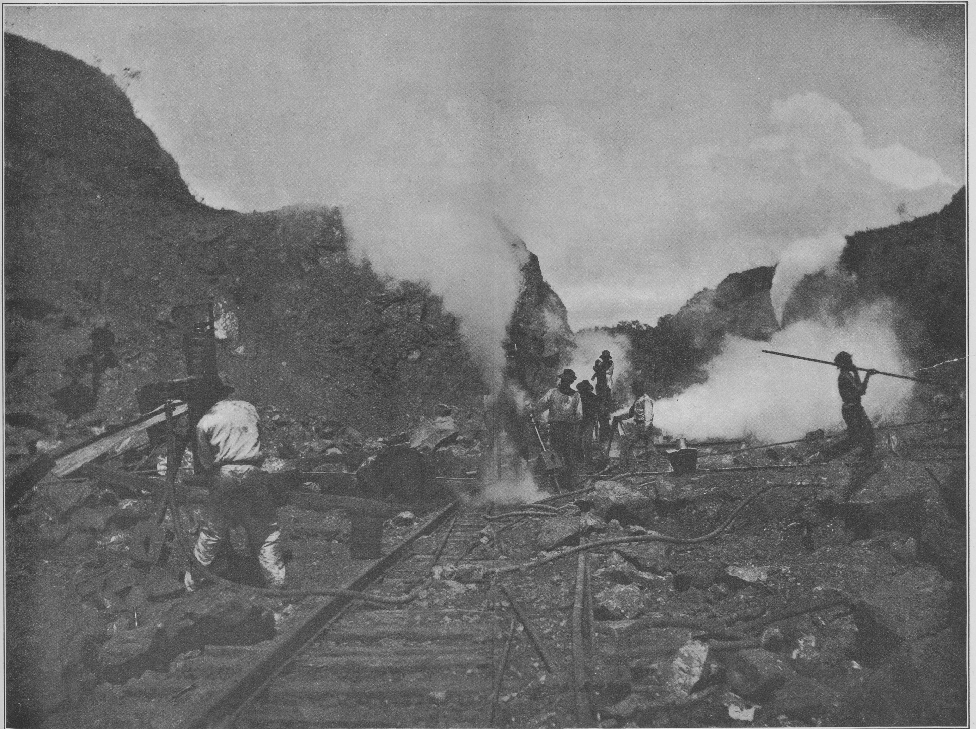
STEAM DRILLS AT WORK IN BAS OBISPO CUT.
