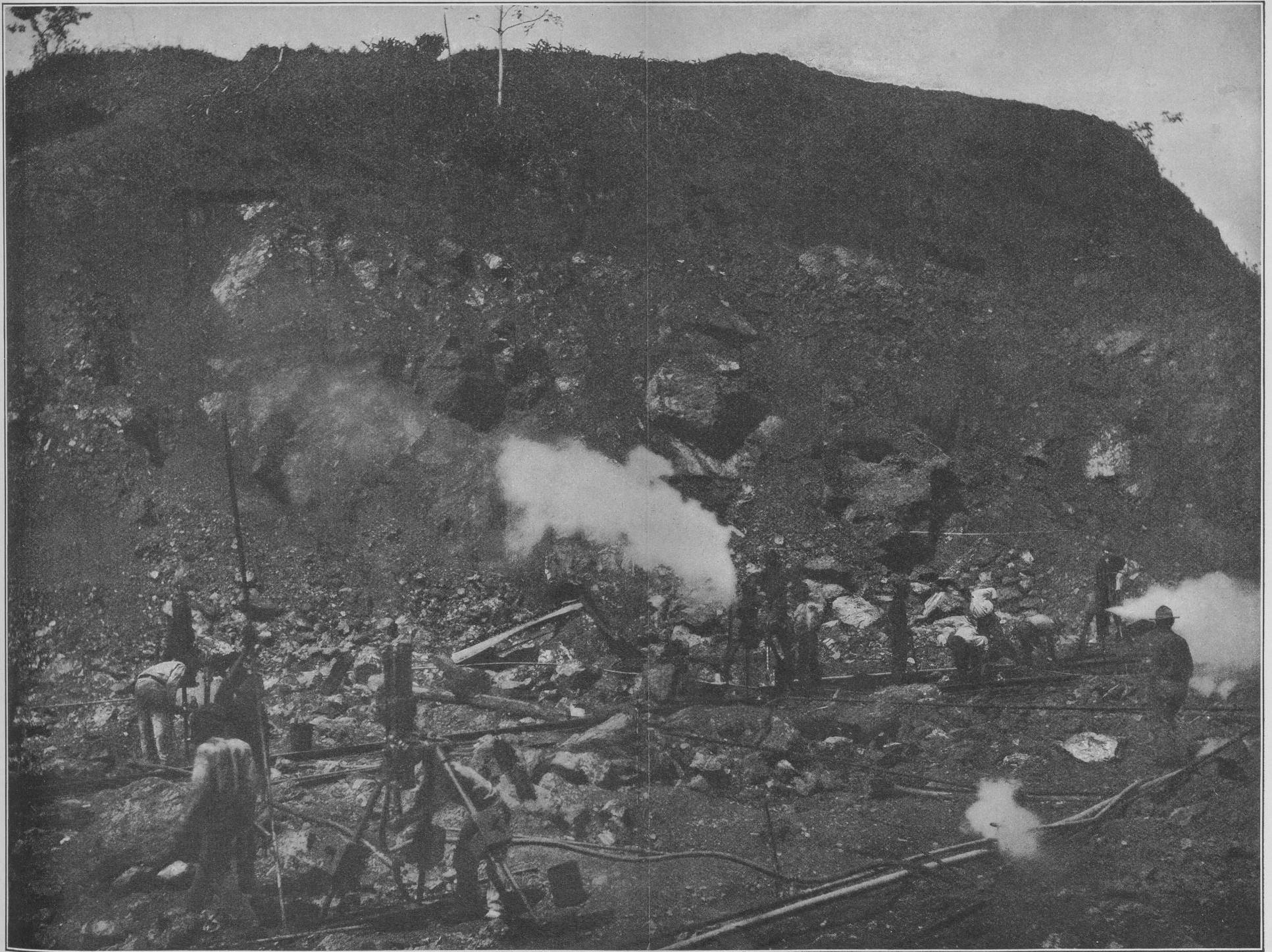
ANOTHER VIEW OF STEAM DRILLS AT WORK IN BAS OBISPO CUT.
