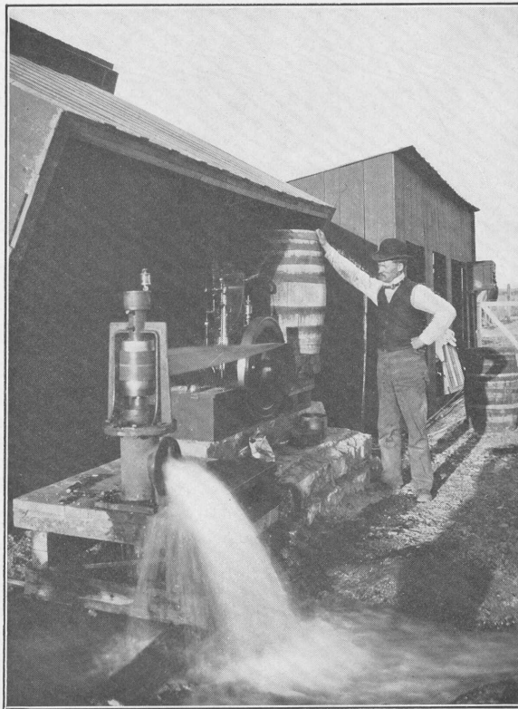
B. SHERMAN'S PUMPING PLANT, NEAR ROSWELL, N. MEX.
