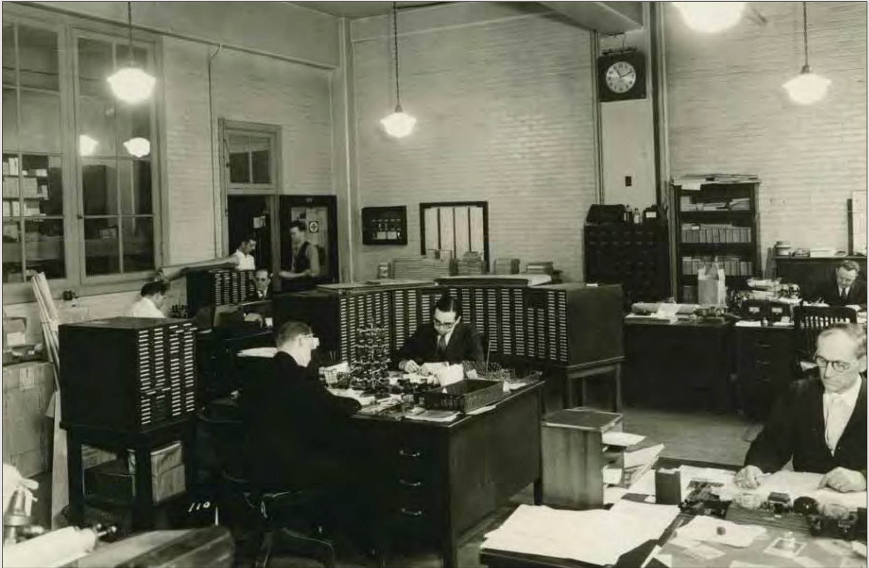
Recordkeeping and accounting for materials was a massive clerical task. The clerks at the center in this photo from the 1930s are using a “Kardex” file, a system for “visible indexing” that paved the way conceptually for later machine assisted systems.
