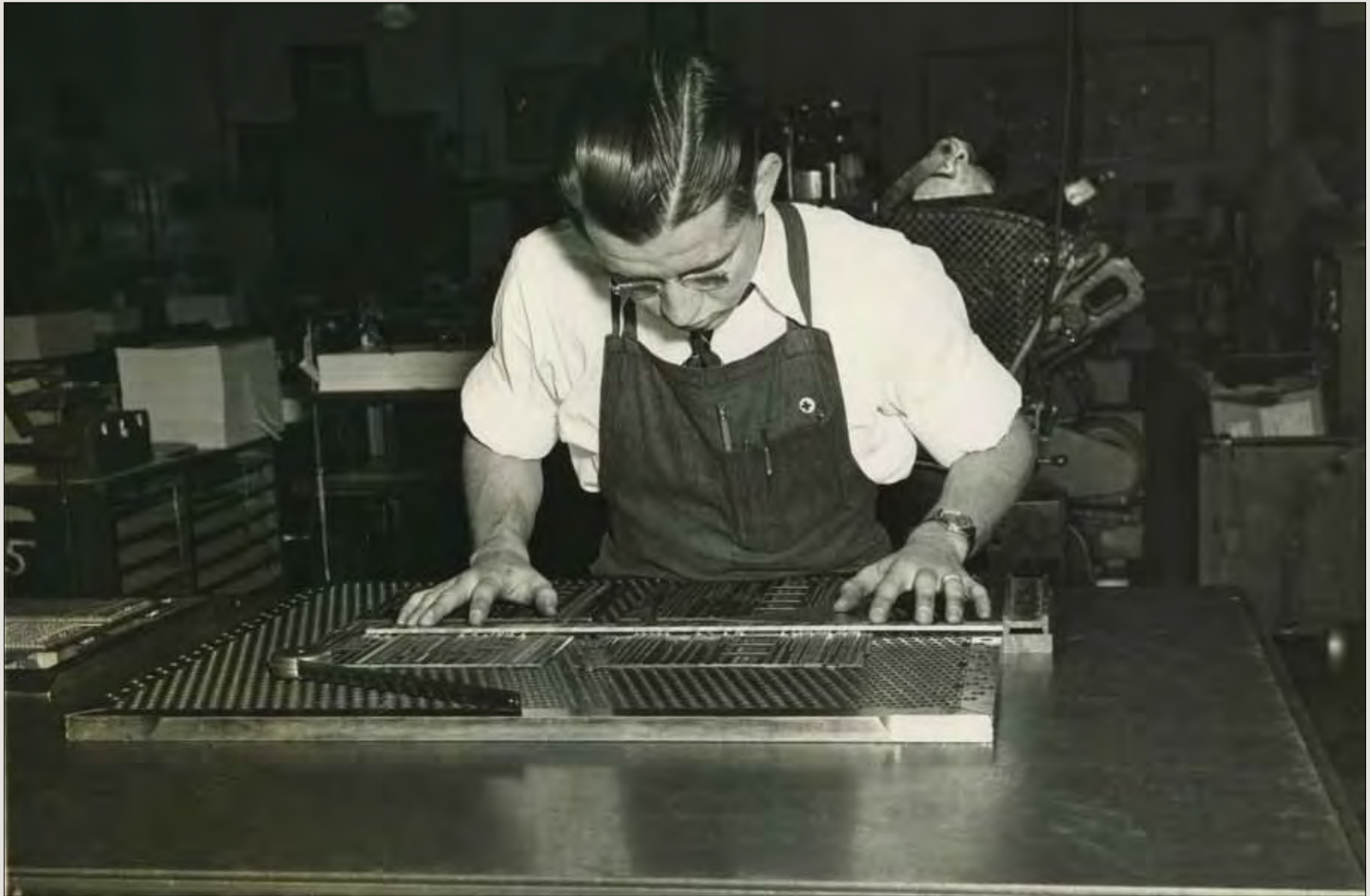
Electrotype plates are imposed into page forms.
