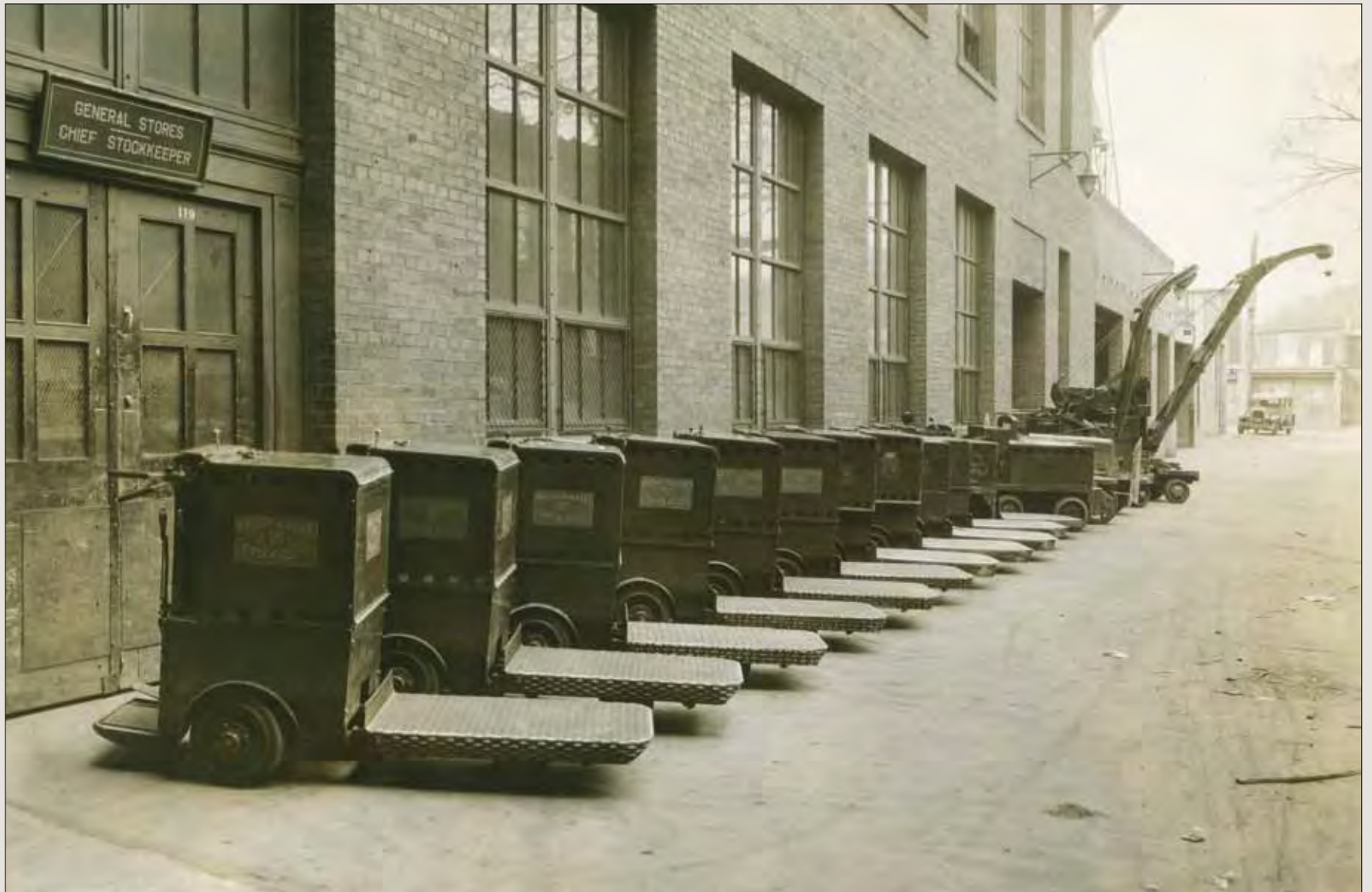
Various kinds of trucks, tractors, cranes, and lifters were used to move and stack heavy materials around GPO's plant. These electric tractors were used for moving paper and product during the 1920s.
