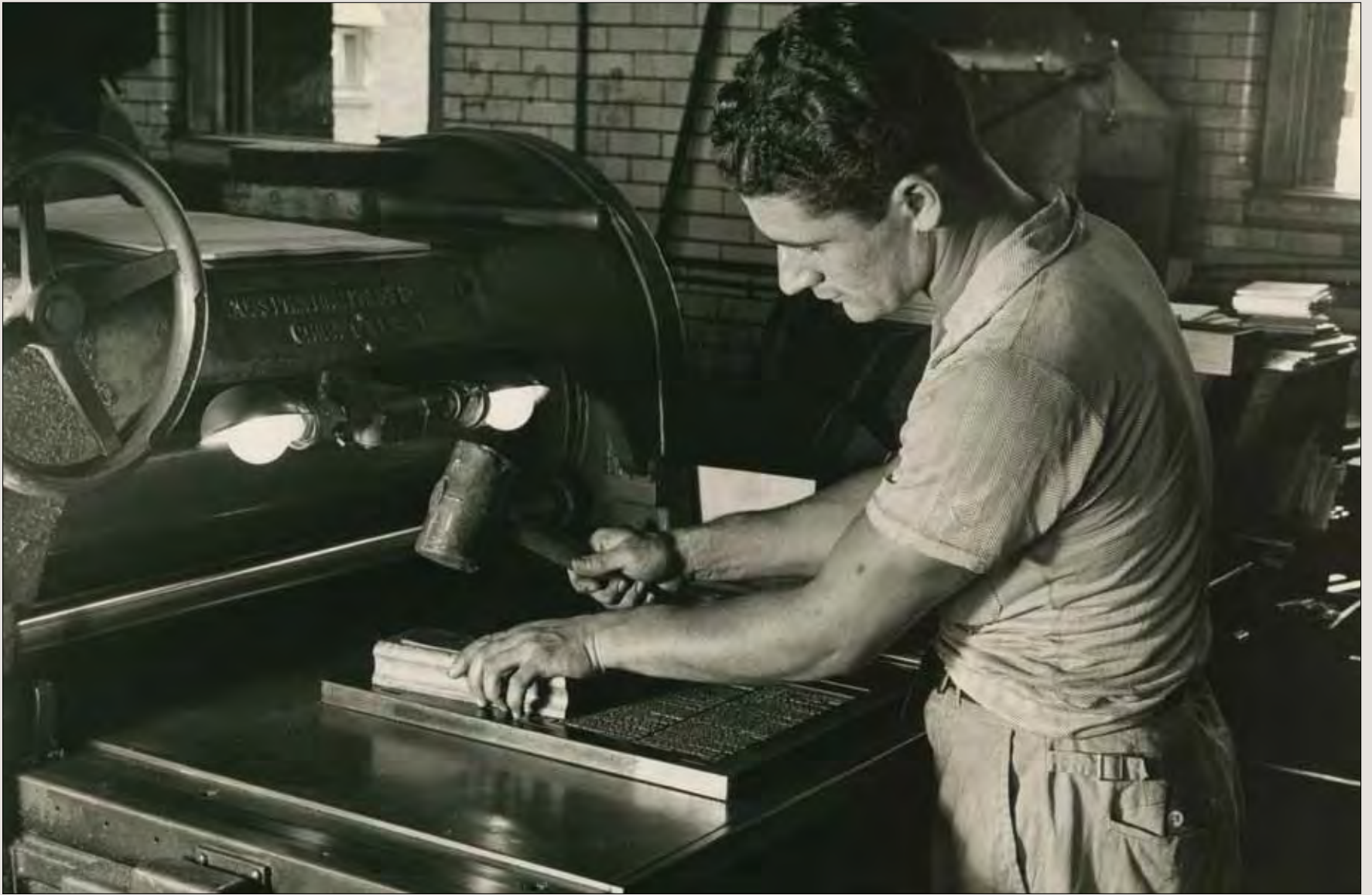
In the 1930s GPO was still primarily a letterpress shop, but a variety of platemaking techniques were employed for various classes of work. Here an apprentice adjusts a chase of type for height before taking an impression for the casting of an electrotype plate
