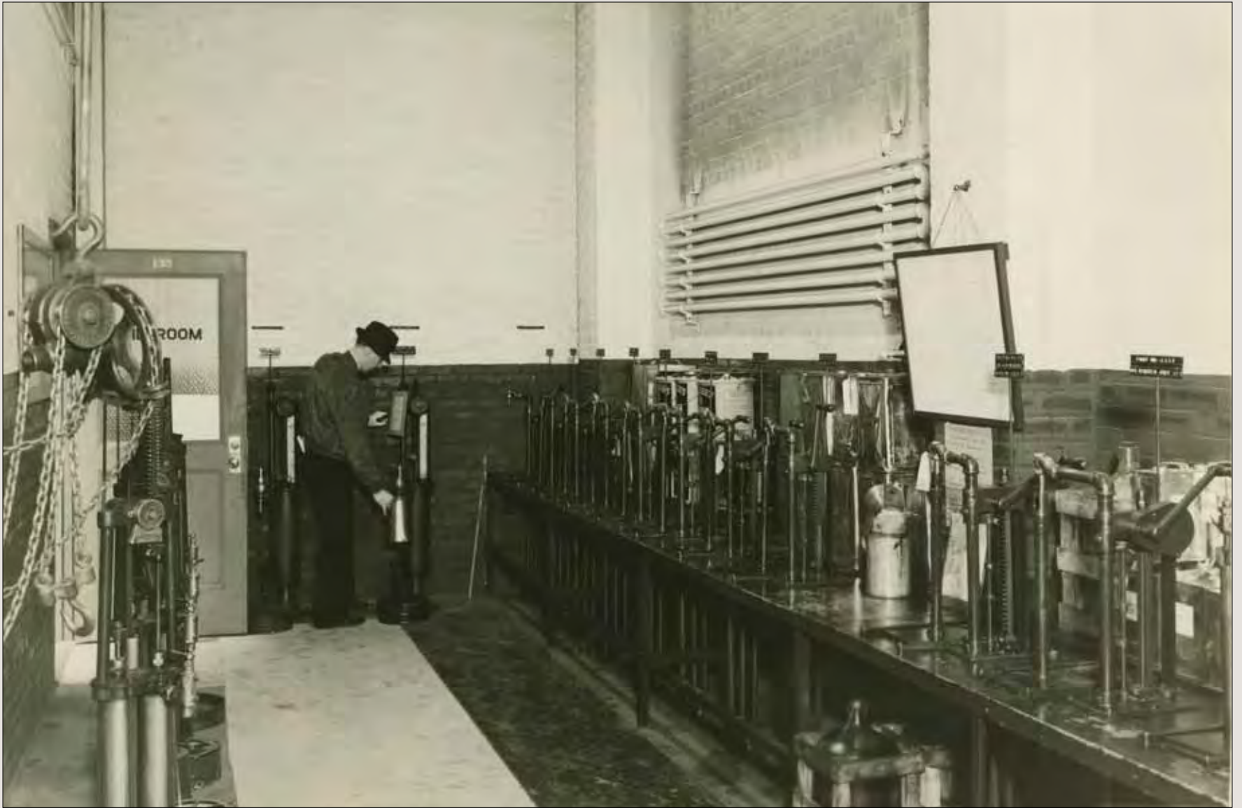
Printing called for a variety of solvents and lubricants. In this photo from the 1930s, these pumps delivered gasoline, kerosene, and other solvents.
