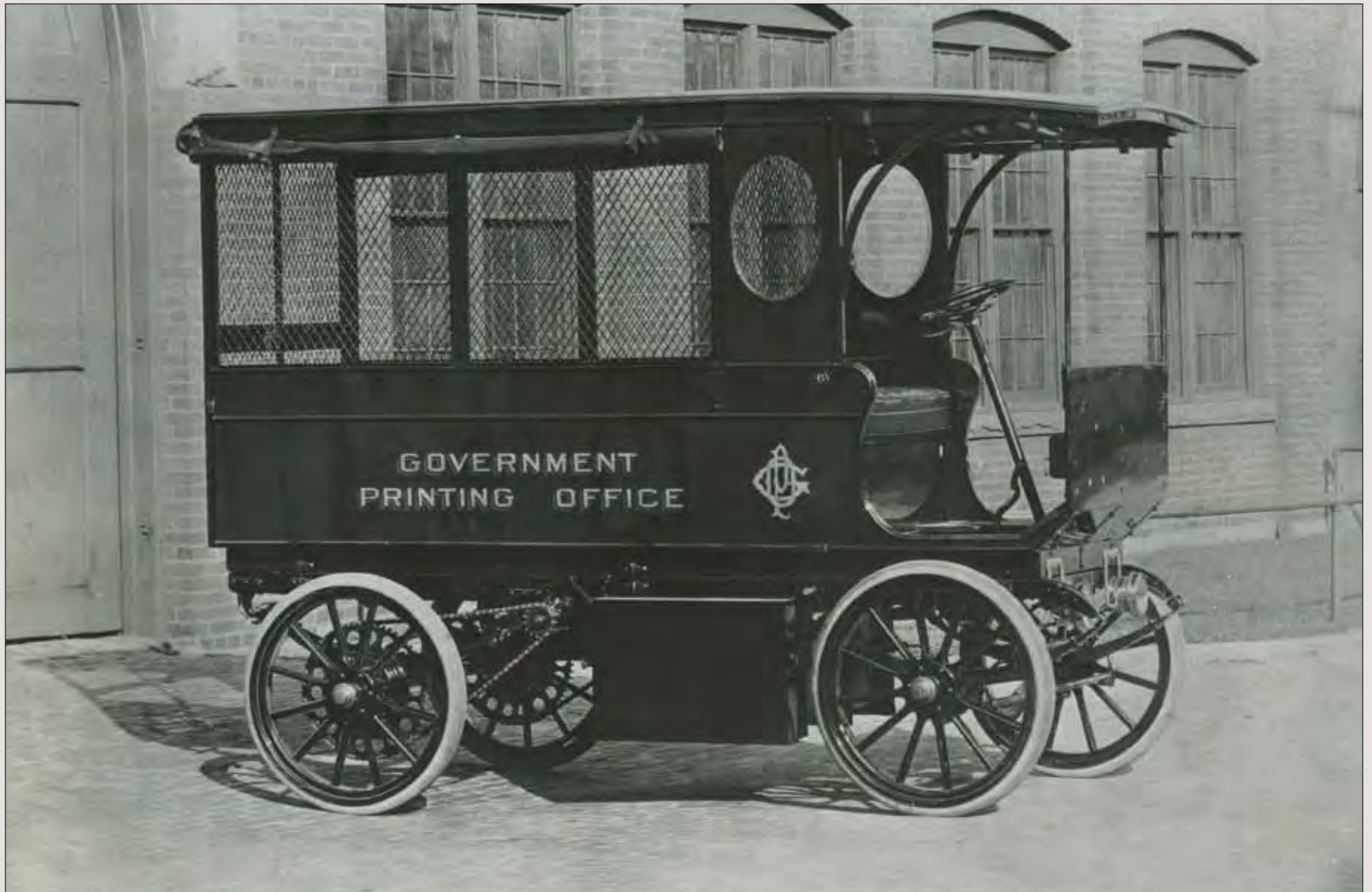
Automobiles came to GPO in 1912 in the form of Baker Electric trucks, manufactured in Cleveland, Ohio. The chain-driven trucks ran on large, heavy batteries and had more in common with the wagons they replaced than with later automotive design.
