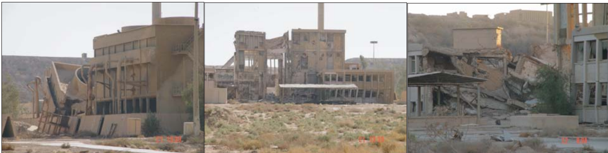
Building 17: Tammuz/cooling tower (Osirak) (left and center); Tammuz-2 (ISIS) (right).
