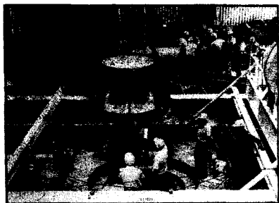
Figure 2.2.6 Rocket Motor Nozzle Assembly — Aerojet Dade Plant NASA-SRM Program, 1964-1966
