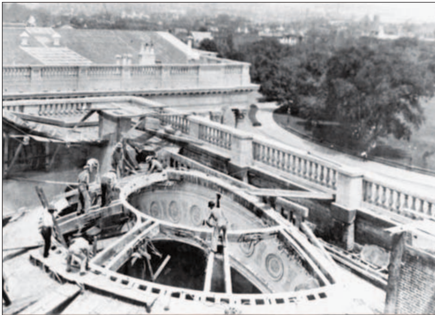
Figure 19. Workmen rebuilding the roof of the Supreme Court ceiling (Old Senate Chamber) in 1901.
