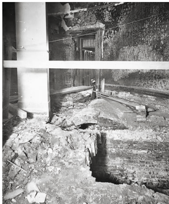
Aftermath of the Gas Explosion 1898
