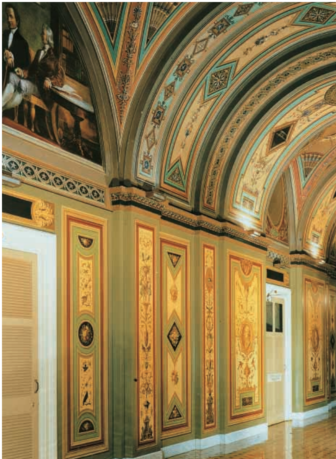
Fig. 15-3. Section of the North Corridor. Overpainting over the years darkened and coarsened the original decoration of the walls, leaving the borders a murky green and the background fields yellow.
