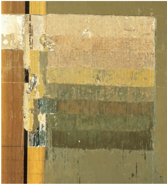
Fig. 15-6. Test window showing the gradual color shift in overpaint. This scala through layers of overpaint at the edge of the trompe l'oeil molding shows nine major paint layers. They shift from the lowest, original, layer of stony light gray to muddy green. Photo: Cunningham-Adams.
