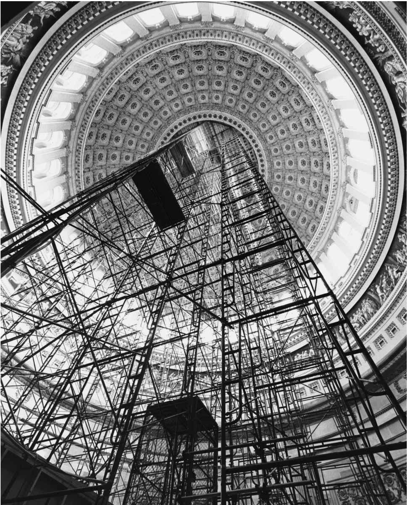
Fig. 13–3. Scaffold constructed for the restoration of the canopy. The 150-foot-high structure supporting a wooden floor at the base of the fresco filled much of the Rotunda for a year.
