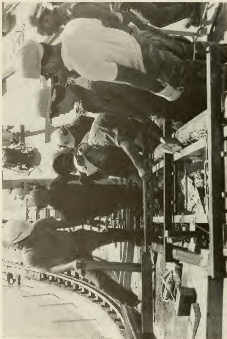
Workers pause as an engineer checks the alignment of the rail during rehabilitation of the locks locomotive tow track. Approximately $100 million of the Canal's annual operating budget is dedicated to maintaining and improving the waterway.
