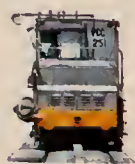
Above: Track shifter at work, Tabernilla Dump, August 13, 1907. This ingenious device, developed by W. G. Bierd, manager of the Panama Railroad from 1905 to 1907, did the work of 250 men.
