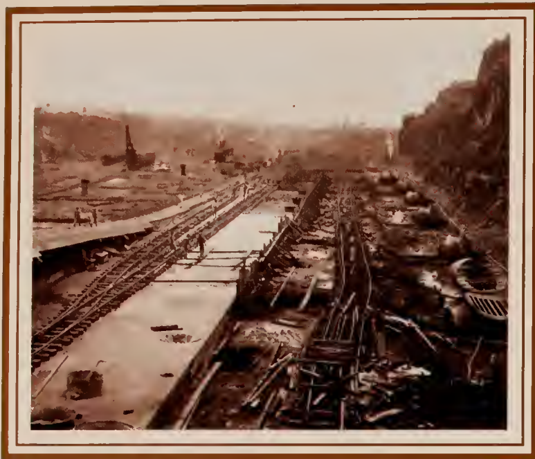
Above: Gatun Locks, July 2, 1910. Visible in the first floor section poured are the 5-foot holes through which water will enter the lock from lateral culverts under the floor. Below: Gatun Locks, April 15, 1911. The 18-foot high main culverts in the lock walls are visible in the completed sections.
