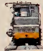
Left: The control board at the locks shows in miniature the position of each gate. The vertical gauges show the height of the water in each chamber.
