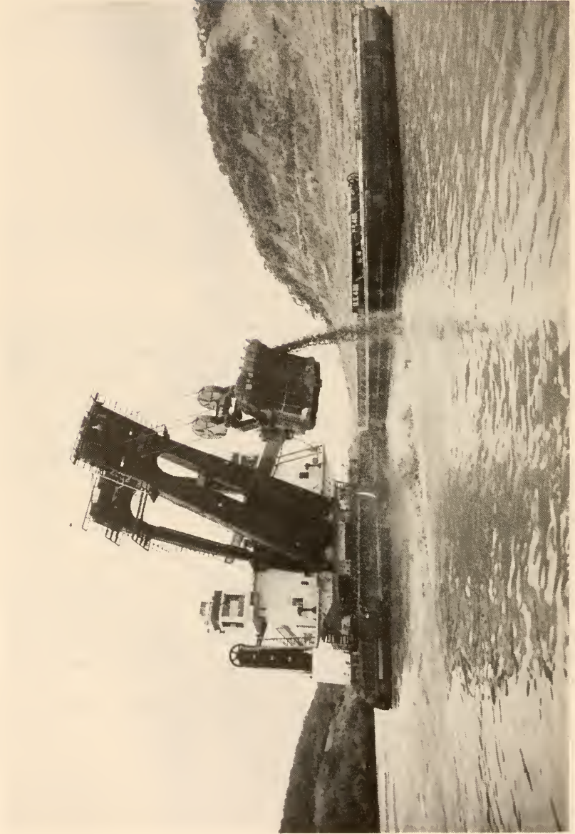
THE DIPPER DREDGE "CHRISTENSEN"—busy at work on the channel deepening project in Gaillard Cut.
