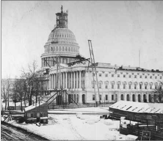
The installation of the Statue of Freedom nearing completion, 1863.
