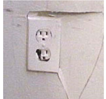
Figure 2: Broken Outlet
