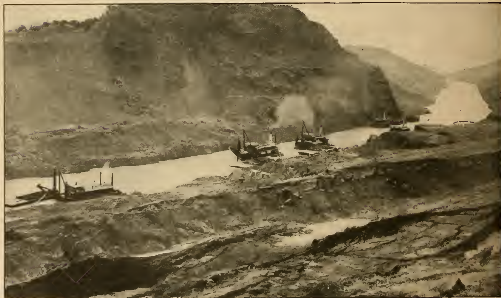
BROKEN-UP CONDITION OF WEST BANK PRECLUDING STEAM-SHOVEL OPERATIONS.
