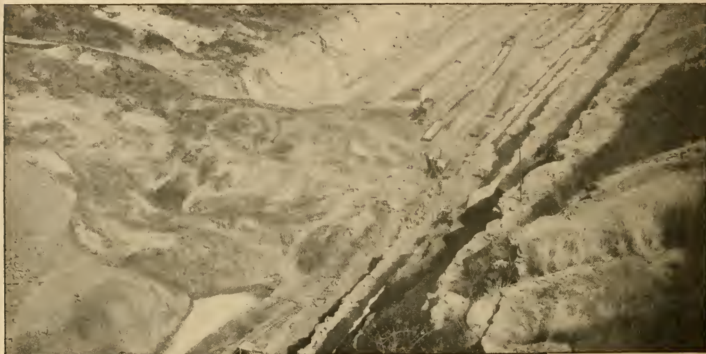
CUCARACHA SLIDE AFTER RUPTURE OF SUPPORTING ROCK MASS.
