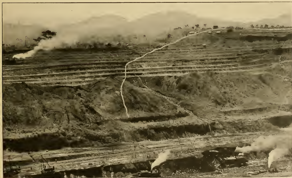
BENCHING ON EAST BANK OPPOSITE CULEBRA (AREA OF BREAK INDICATED).
