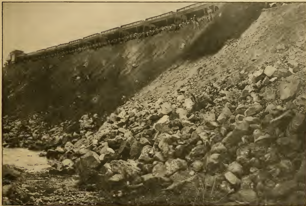
NATURAL SLOPE OF MATERIAL EXCAVATED FROM CANAL PRISM.
