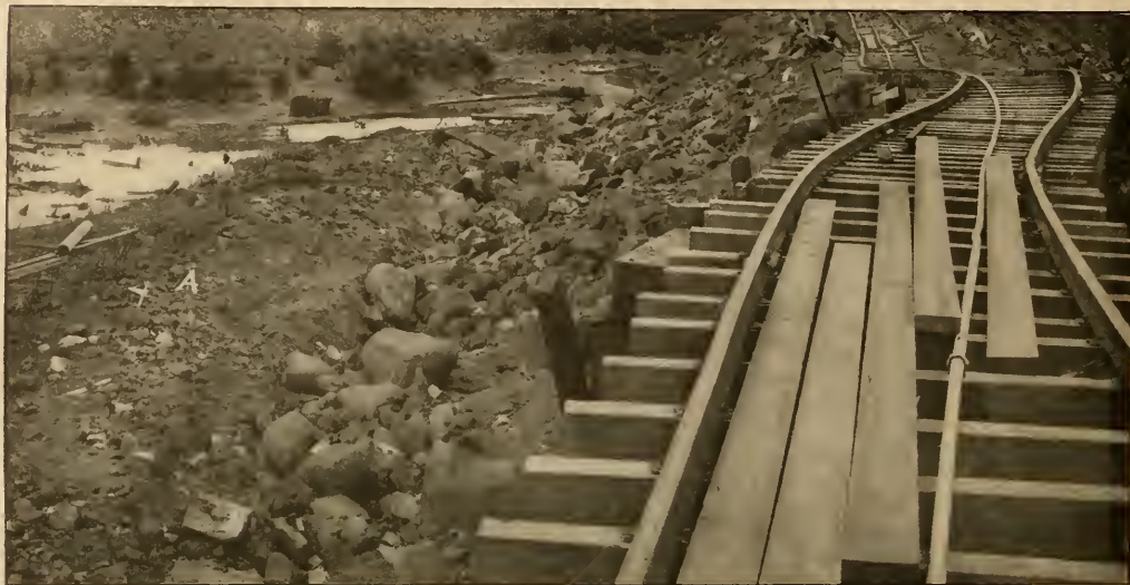
SOFT GROUND "A" PUSHED UP BY WEIGHT OF EMBANKMENT.
