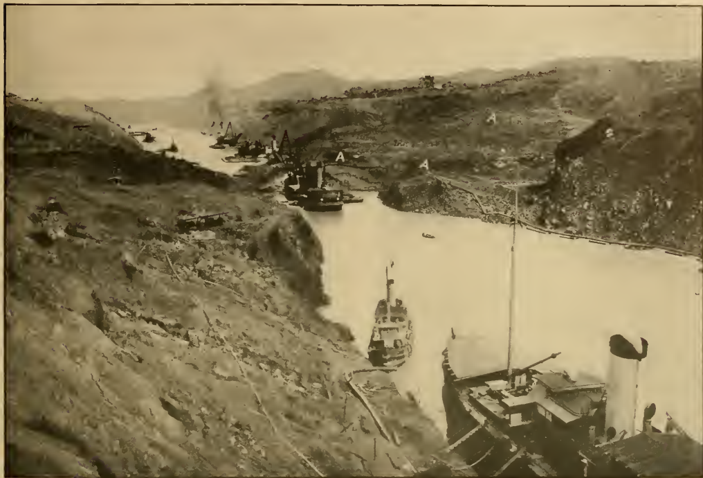
COMPLETE CLOSURE OF CANAL: WAVES THAT ARE MOVING DOWN SHOWN AT "A."
