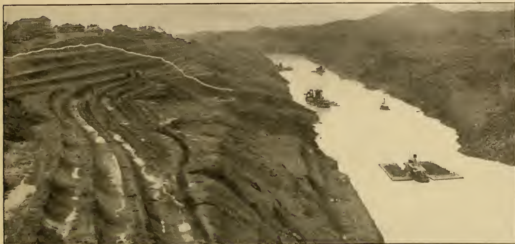
ARRANGEMENT OF BENCHES ON THE WEST BANK NORTH OF CULEBRA (AREA OF PRESENT BREAK INDICATED).
