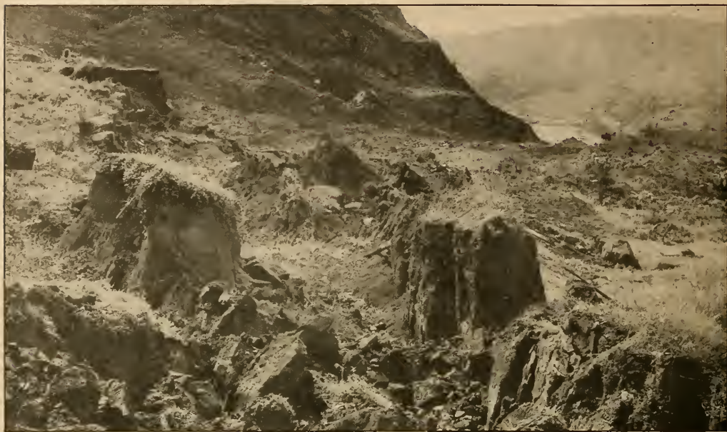
BROKEN-UP CONDITION OF EAST BANK PRECLUDING USE OF STEAM SHOVELS.
