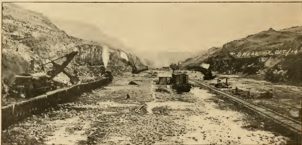
SECTION OF CANAL NOW BROKEN DOWN, AS STEAM SHOVELS WERE COMPLETING EXCAVATION OF PRISM; HAGAN'S SLIDE IN DISTANCE, SUBSEQUENTLY REMOVED BY DREDGES.
