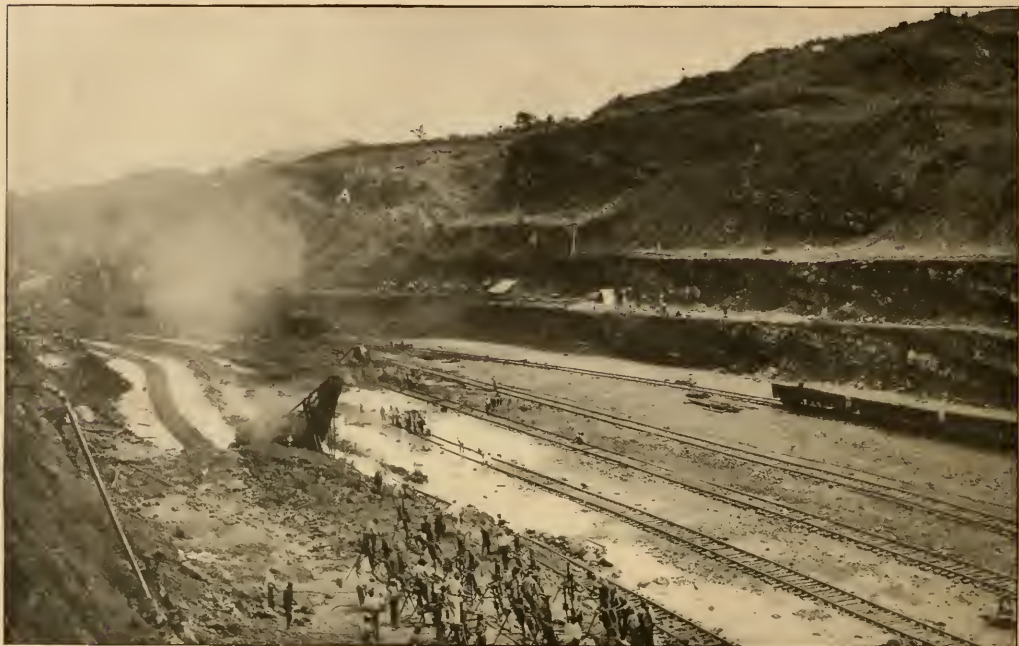
SHOVELS REMOVING FINAL BENCHES IN VICINITY OF CULEBRA; HAGAN'S SLIDE AT "A."
