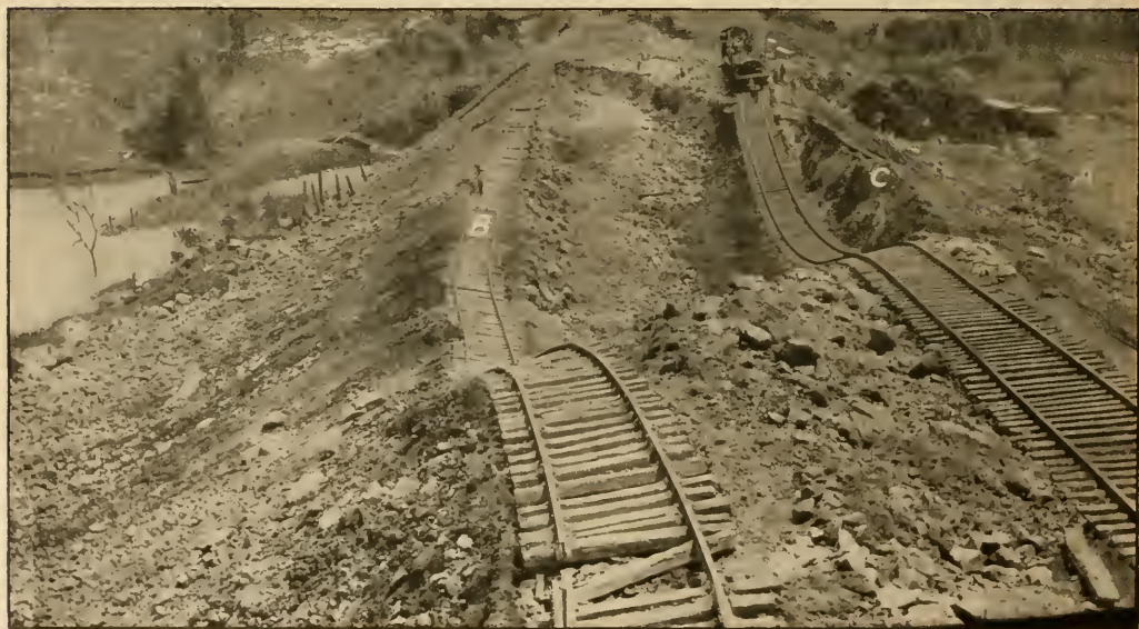
WEAK UNDERLYING STRATA PUSHED UP "A" BY WEIGHT OF EMBANKMENTS "B"; SPREAD "C" NOT SUFFICIENT TO PRODUCE EQUILIBRIUM.
