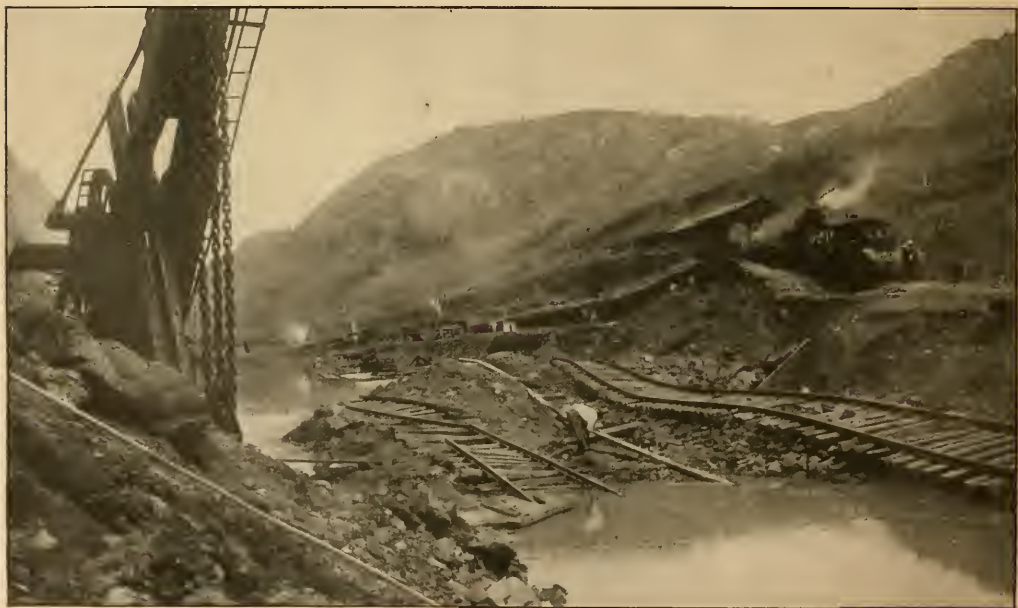
UPHEAVING OF BOTTOM AND EFFECT OF A BREAK IN THE PRISM DURING DRY EXCAVATION.
