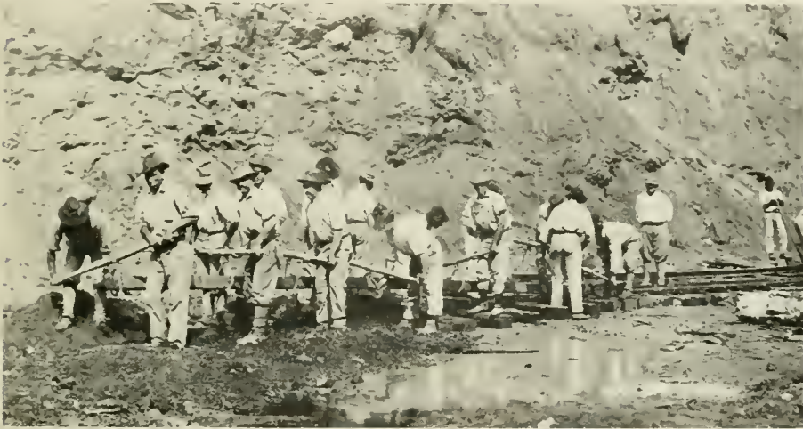
Spanish workers remove tracks from Culebra (now Gaillard) Cut in 1913 before water is let into the Canal prism.
