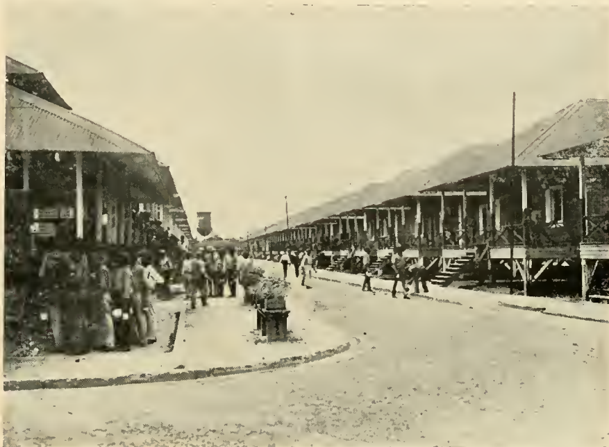
CAMP BIERD, where there is now only a house or two and a cluster of bachelor barracks, was once the bustling town shown in this old picture. The men in the foreground are lined up at the messhall.
