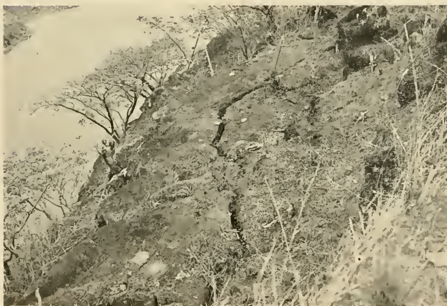
THE CRACK—a threat to the precipitous hill
