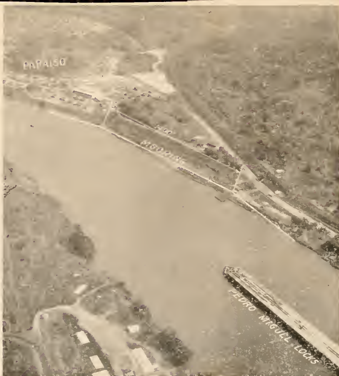
Mooring facilities for two big ships north of Pedro Miguel Locks would reduce congestion and increase Canal capacity during Pacific Locks overhaul periods.
