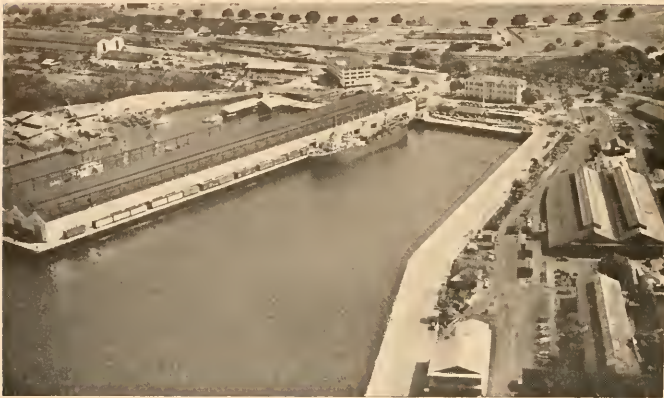
BALBOA'S inner harbor, seen from a plane, shows Pier 18 protruding over 1,000 feet into the quiet water. On the right are Docks 14, 15, and 16, separated by a launch landing from the completely shielded pier. The line of railroad cars on Pier 18 shows part of the cargo handling facilities available.
