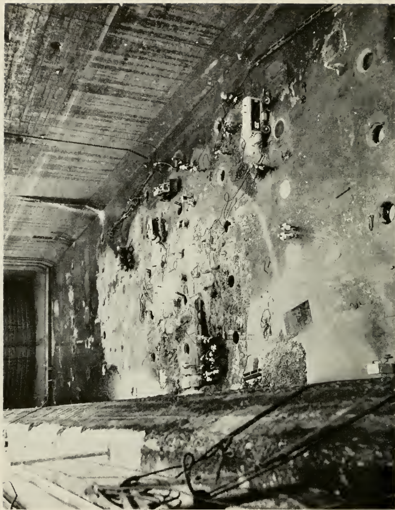
Repairing Culvert Failure in East Chamber, Pedro Miguel Locks.
