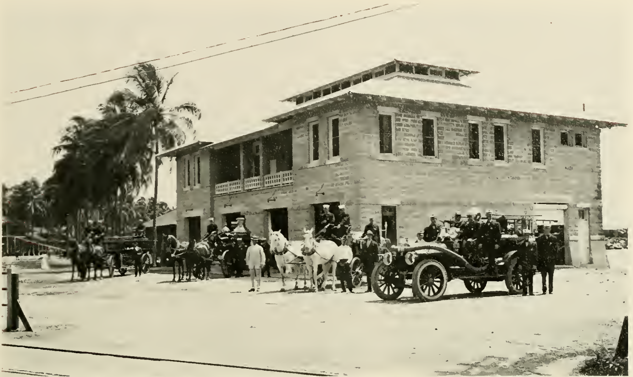
A new reinforced concrete fire station at Cristobal was completed in August, 1912, and motor equipment was on order to replace the remainder of the horse-drawn engines.
