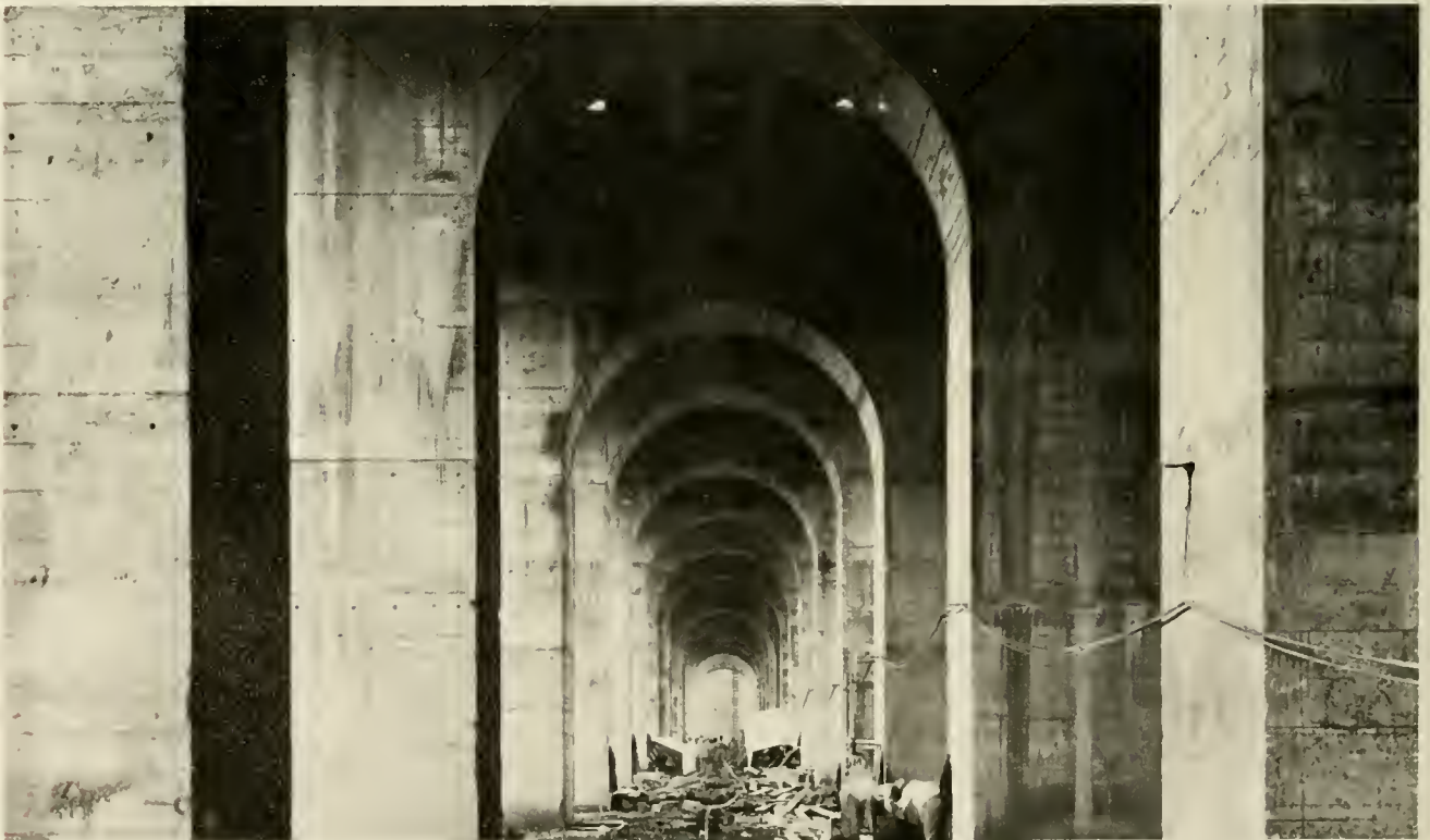
Just 14 months before the Canal opened, this interior view of the north approach wall to Gatun Locks resembled a stark cathedral, stripped of all statuary and religious symbolism. At right: An aerial view of Gatun Locks and Gatun Lake.
