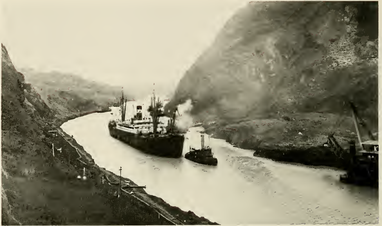
The "SS Ancon" passes a slide in Gaillard Cut during the official opening of the Canal, August 15, 1914.
