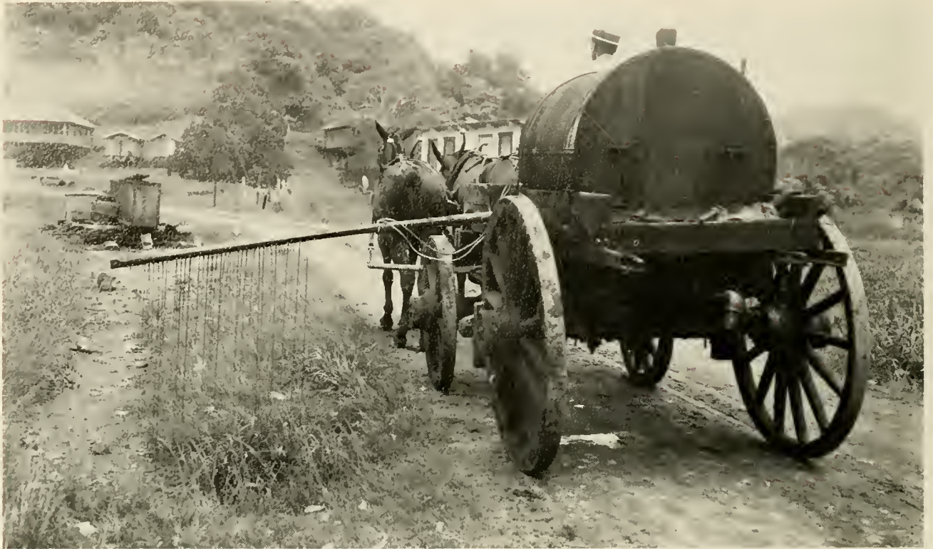
Sanitation played a vital part in the construction of the Canal. Ridding the area of the dread yellow fever and malaria was the responsibility of Dr. William Crawford Gorgas.
