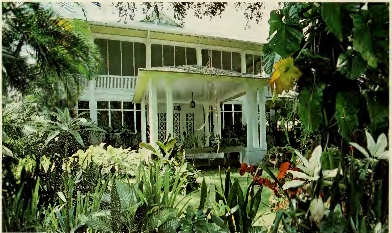
Though renovated and air conditioned, the classic architectural style of the early 1900's, the wide verandas and high ceilings, are still charming features of the Governor's House as it appears today.
