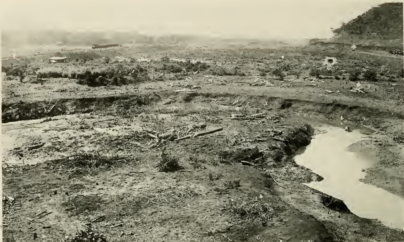
In October 1908 work had scarcely begun on the desolate swampland that would one day be Miraflores Locks.
