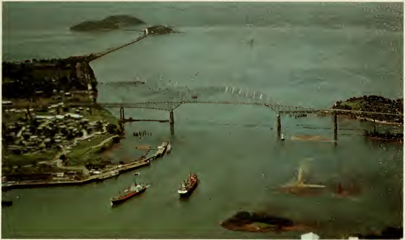
Built at a cost of $20 million, the bridge was inaugurated on Columbus Day, October 12, 1962, in a ceremony attended by Panama and U.S. Government officials and diplomatic representatives.
