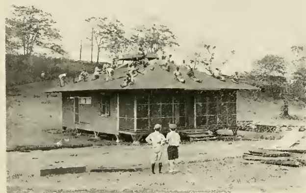
Houses were dismantled and moved to new locations.
