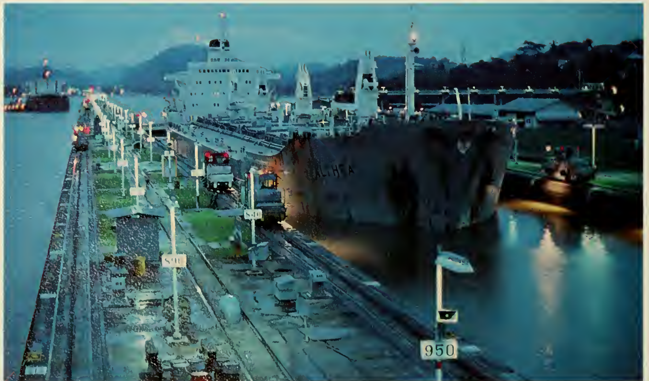
Moving through Miraflores Locks, the "Althea" produces a dramatic night scene. An elaborate lighting system makes it possible for the Canal to operate 24 hours a day.
