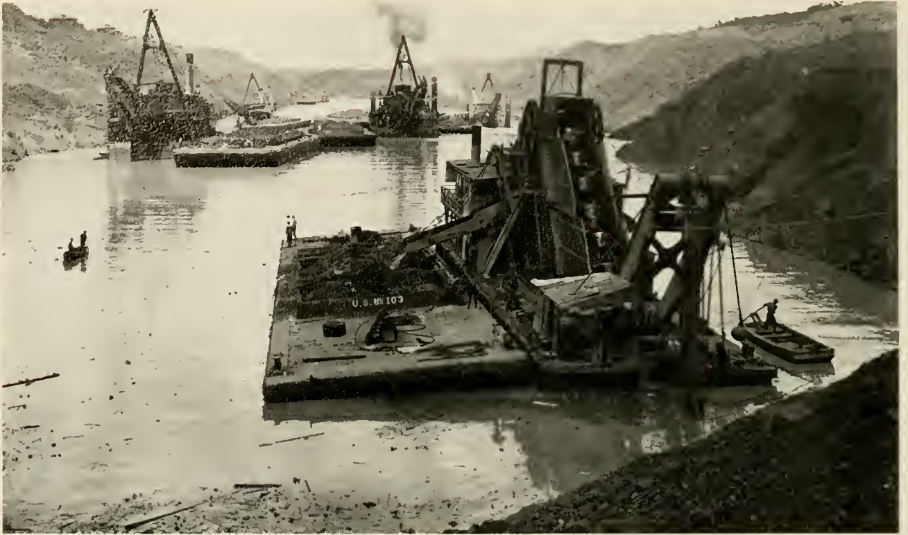
The Panama Canal's fleet of dredges scooped out tons of rock and earth from the newly named Gaillard Cut after a slide in September, 1915 closed the Canal to traffic for seven months.
