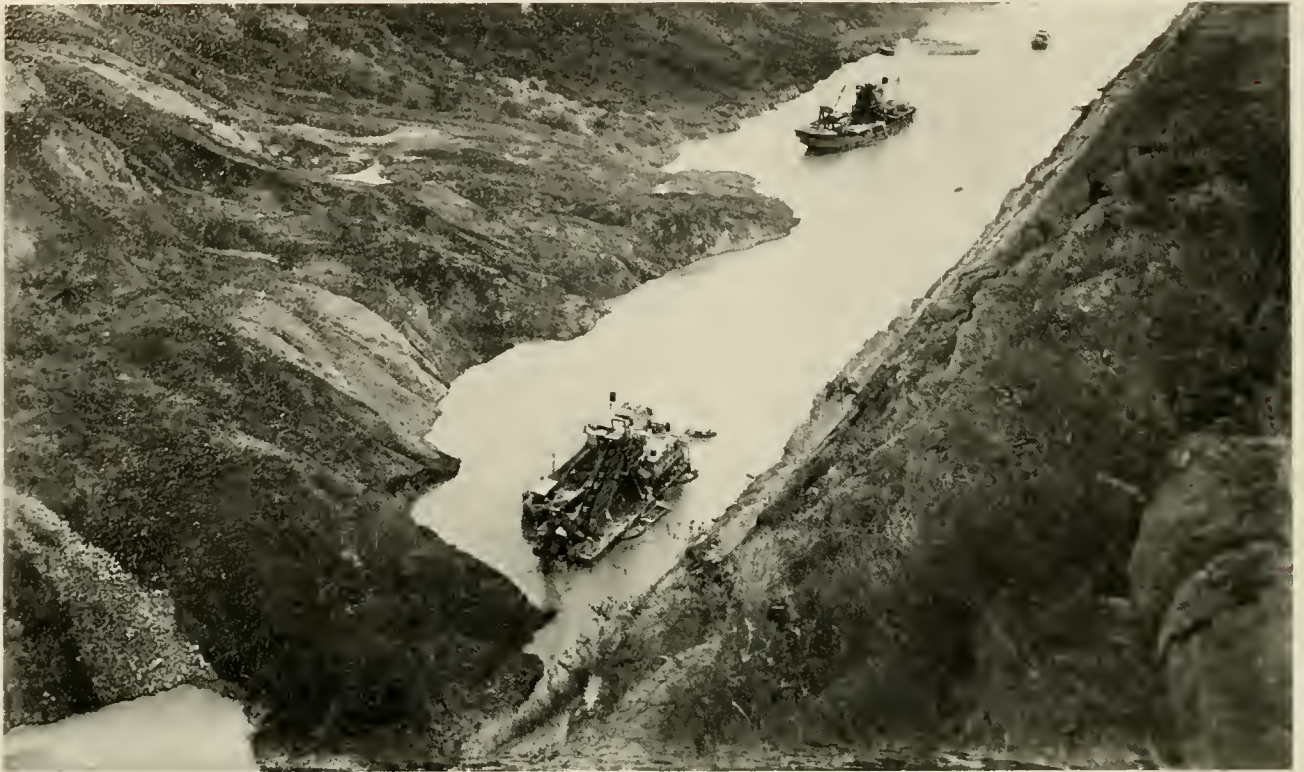
Devastating slides, such as this one on December 3, 1913, plagued the Canal during its construction and continued after the Canal was opened. An avalanche, September 15, 1915, closed the Canal for seven months.
