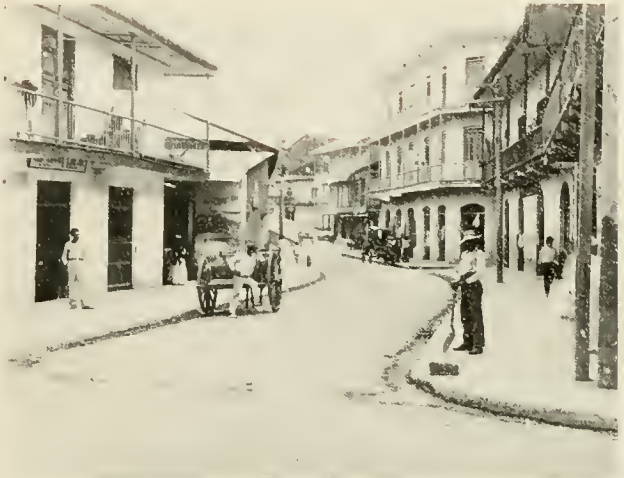
Here is the same street after paving, two months later.
