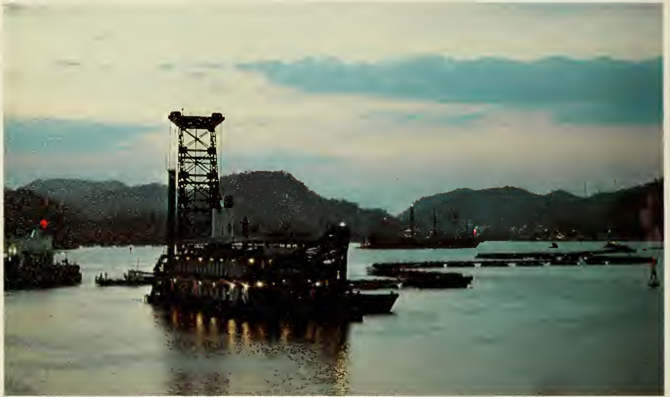
The lights of a suction dredge glow brightly as work continues around the clock. Continuous dredging is a vital part of Canal operations.
