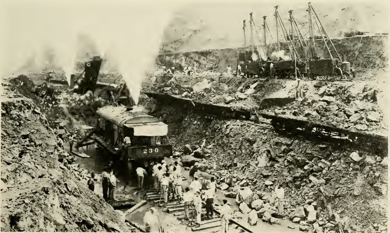
Steam shovels #230 and #222 meet "nose to nose" on completion of bottom pioneer cut at Culebra May 20, 1913. All that remained was to widen it to 300 feet. The many puffs of steam indicate the great activity all along the line at that time.
