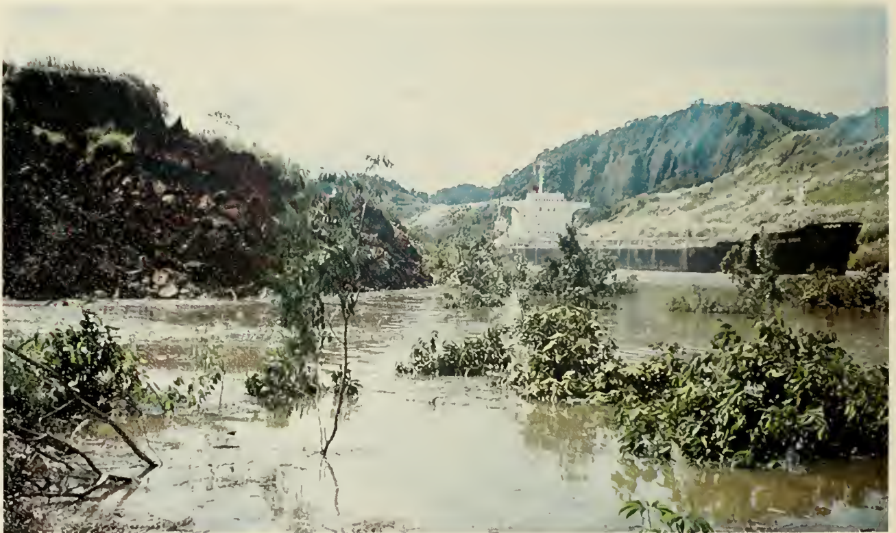
This slide, October 10, 1974, dumped 1,000,000 cubic yards of dirt along with trees and shrubs into the Canal channel.
