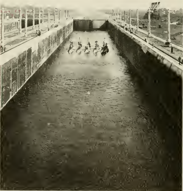
Guided with hand-held lines instead of towing locomotives, these vintage submarines resemble toys in a huge bathtub as they make their way into the locks which were sometimes used as dry docks before the Canal was officially opened.
