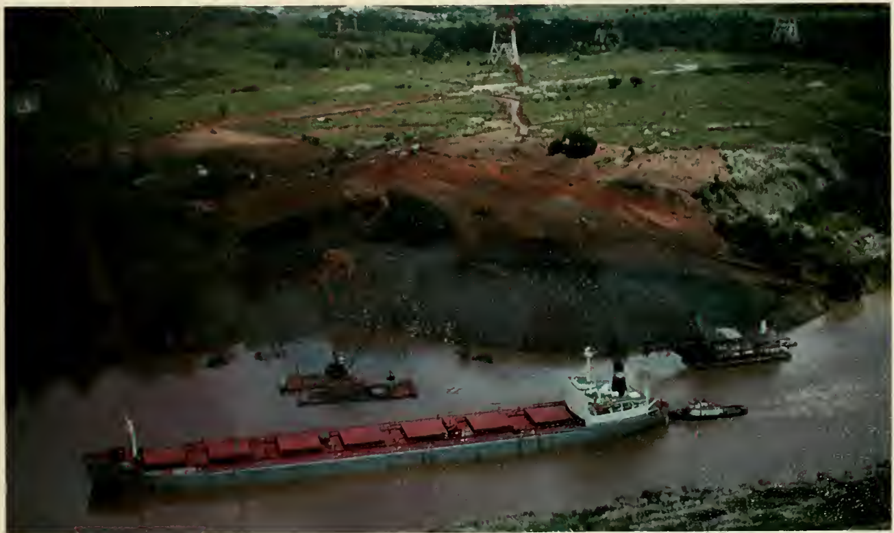
A large vessel maneuvers carefully past the slide with the assistance of a tug. The Canal was closed for several hours while hydrographic survey crews determined that half of the channel could be used for one-way traffic.
