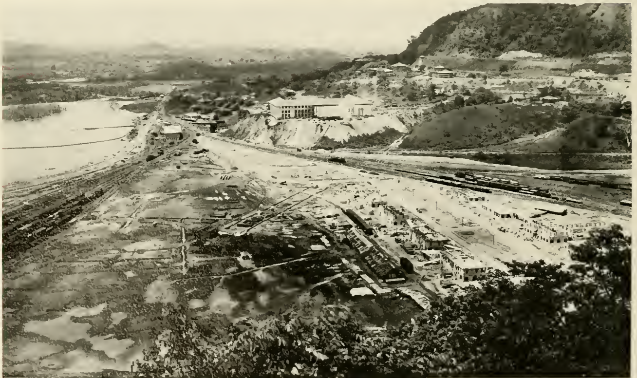
Two years later, in May, 1914, one wing of the Administration Building had been completed and work was progressing on the employee quarters along the street that was to be named the Prado.
