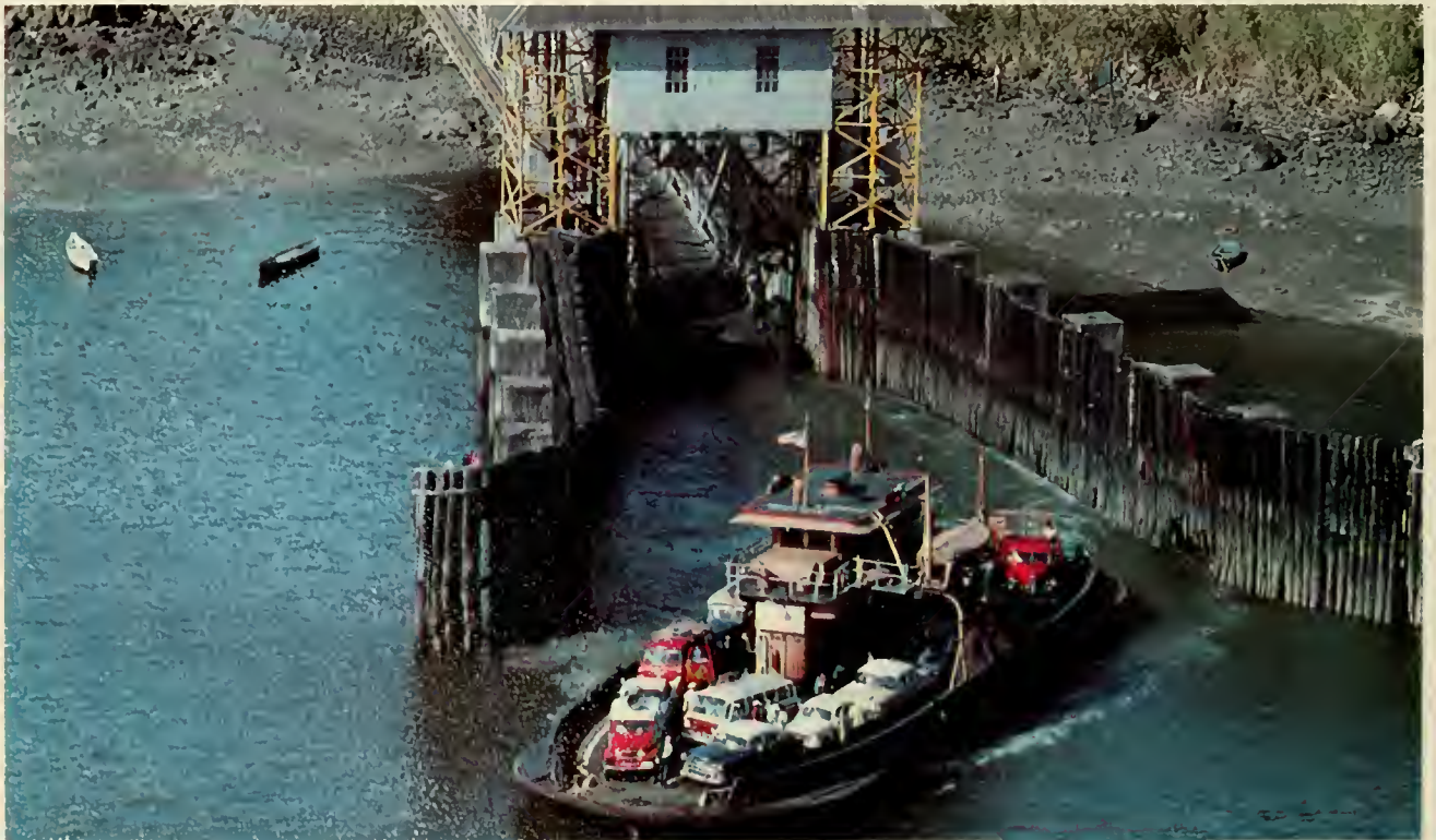
The ferry continued to operate, carrying passengers and vehicles across the Canal until October, 1962, when the Thatcher Ferry Bridge, one of the largest steel arch bridges in the world, was dedicated.
