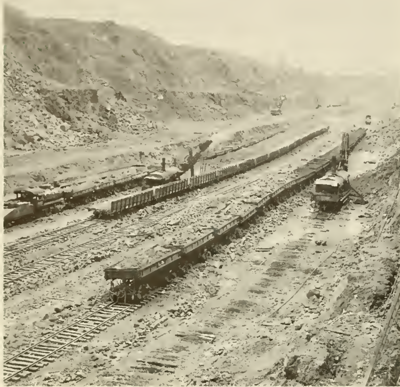
All of Hallen's photographs are carefully identified on the glass plates. The one at left is labeled, "Culebra Cut—Looking south from Cunette. Locomotive No. 607 with train and steamshovel working on bottom of Canal, November 6, 1912." The one below is precisely identified as "Operation of Gatun Locks. Crowd on walls and lower guard gates watching water entering the west chamber of lower locks. View looking south from forebay, September 26, 1913."
