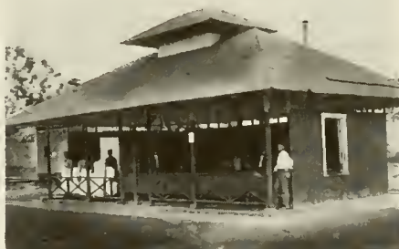
One of the new mess halls at worksite.
