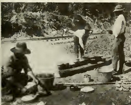
Workmen cooking beside the railroad track.
