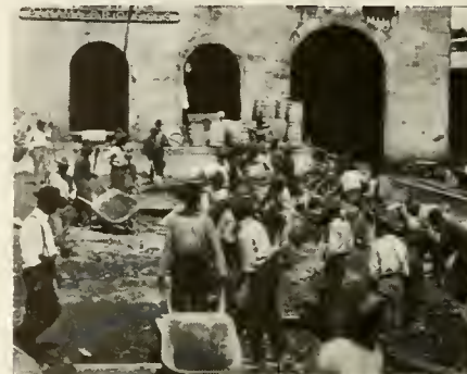
Laying brick at Railroad Station.
