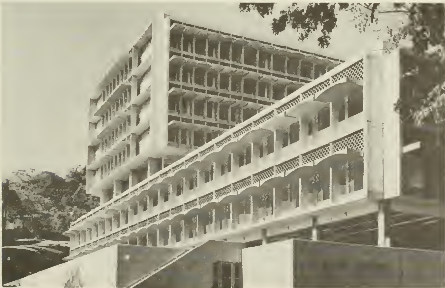
The new Gorgas Hospital annex, the highest and the newest building in the Canal Zone, was put into operation in February 1965. Alterations to the existing plant and construction of this new 8-story air-conditioned building were made to consolidate all Gorgas Hospital activities into four buildings connected by two pedestrian bridges and a tunnel. Sections A and B, two areas devoted to the care of internal medicine patients, were remodeled in 1969 at a cost of more than $1 million. Remodeling of Section O, which will house the pediatric ward and several other units, is scheduled to be completed in 1970.
