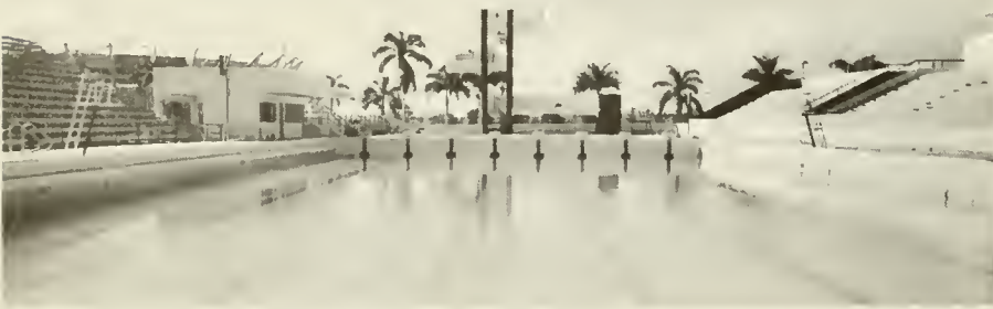
The new $1 million Olympic Pool constructed specially for the XI Games has a capacity for 3,000 spectators to view the swimming competitions.
