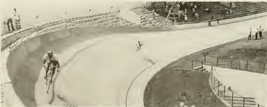
Olympic cyclists take a practice run around the Velodrome near Tocumen Airport. The Velodrome has a 250 meter ring and a cement track with an inclination of from 12 to 45 degrees. Approximately 2,500 cycling fans can watch the races.
