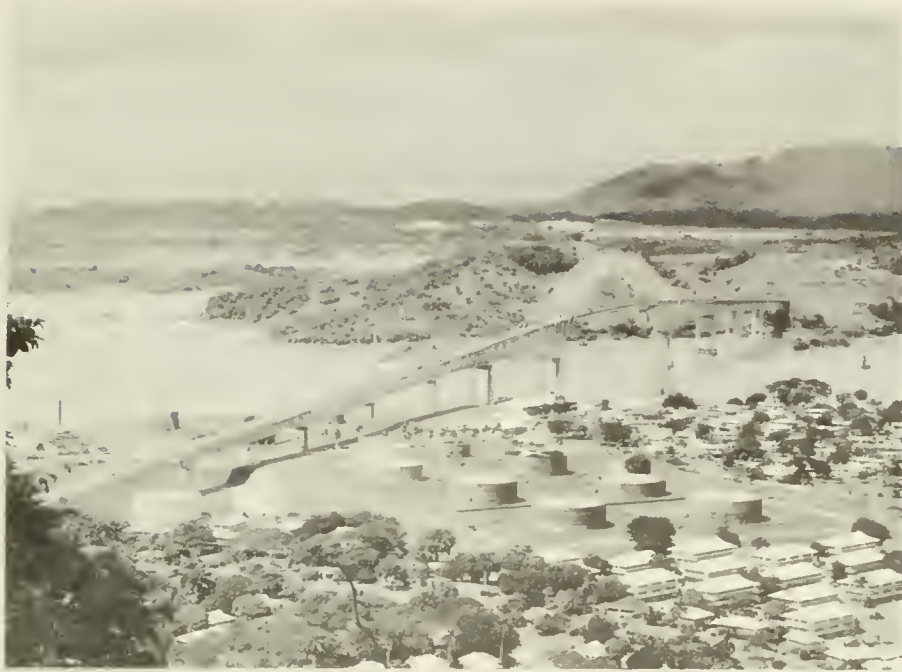
On October 12, 1962, the new $20 million Thatcher Ferry Bridge was dedicated and used by traffic for the first time. Soaring 201 feet above the Canal channel at Balboa at high tide, the bridge is among the highest in the world over navigable waterways. It unites two parts of Panama and two continents and is a link in the Inter-American Highway.
