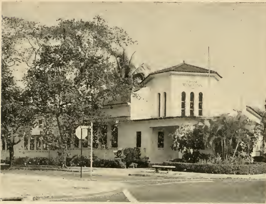
CHASE MANHATTAN's Balboa branch stands at the corner of Balboa Road and Barnebey Street, on the site of the old Balboa Post Office. First occupied in August 1940, it was later enlarged.
