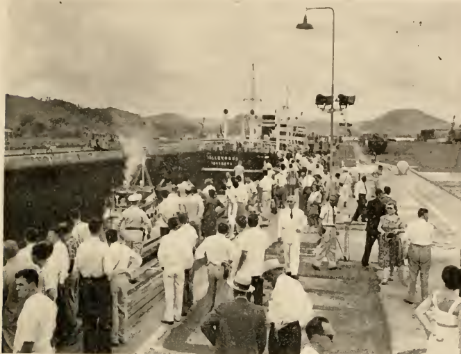
Both waterways and highways carry heavy traffic, although of different kinds, delegates to the recent Road Congress discovered during a visit to the Locks.
