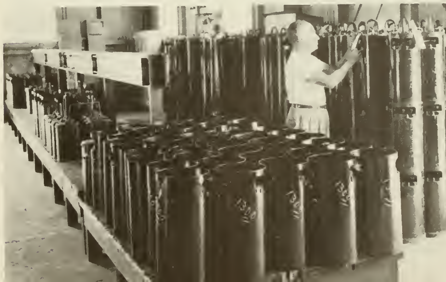
Julio Collazos, electrician, with a bank of re-charged batteries ready to be placed in buoys and beacons. Each charge lasts up to a year to 14 months and some of the batteries have been in use for as long as 16 years.
