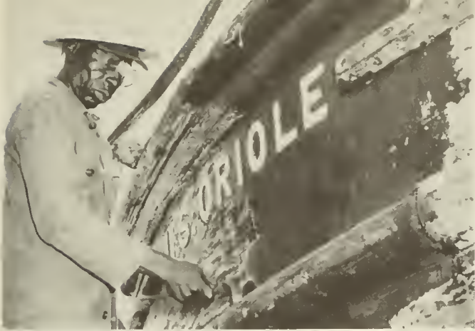
Paint scraping is part of the work at the Launch Repair Shop. Here veteran employee James Miller works on the Oriole, a Balboa launch which is undergoing extensive repairs at Gamboa.
