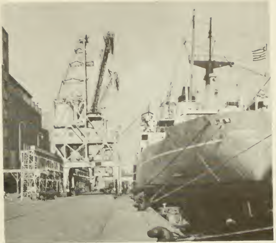
The wheat wharf where stevedoring operations are being carried out. Wheat is sucked up by pipe and sent into the silo at the extreme left.
