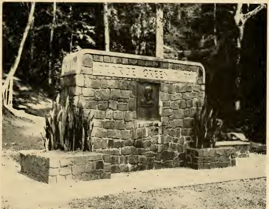
BACKED BY a slender waterfall which tumbles down a steep rock face, George Green Park is dedicated to the memory of the man who was the Canal's Municipal Engineer for over 25 years. It is located on Madden Road; the little park was one of his favorite spots. The monument itself is made from stone from Sosa Hill Quarry and was designed by Leo C. Page of the Architectural Branch. Funds to build it were contributed by Mr. Green's friends and associates. The memorial was dedicated in January 1951.
