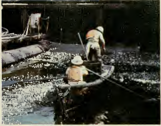
A panga is used for the cleanup job, as boatmen pick up oil-soaked polyurethane foam and deposit it in a drum.
