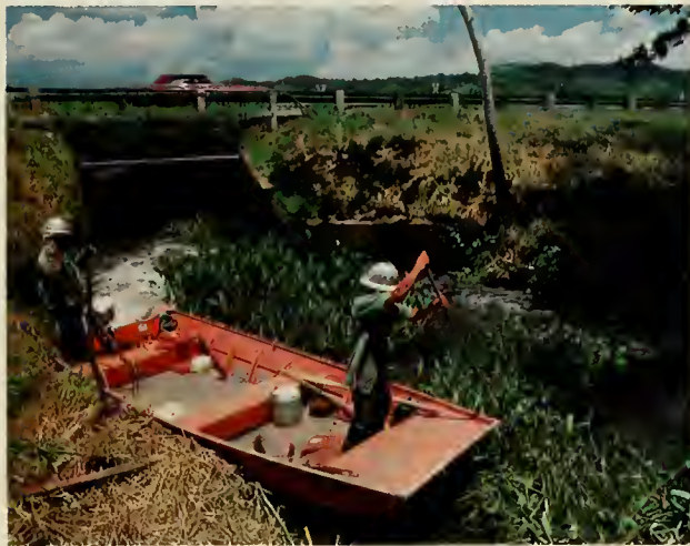
With the additional current provided by an outboard motor, water hyacinths are herded through culverts under Gaillard Highway to a pond for harvesting.
