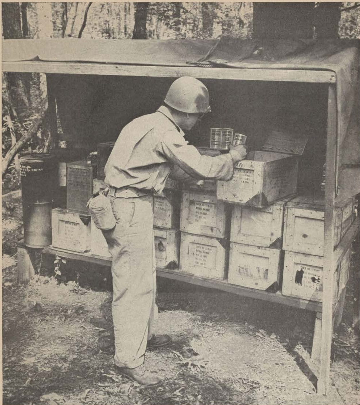
Figure 9. Field storage of methyl bromide in cans. Canvas shelter protects cans from sun and weather.
