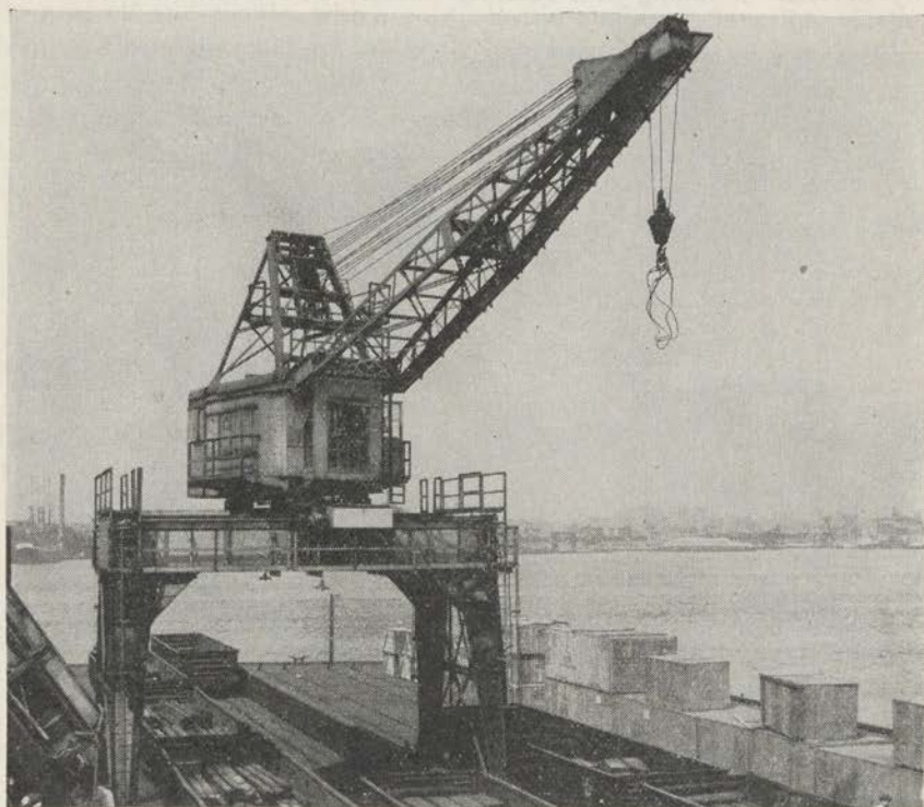
FIGURE 31.—Heavy duty crane, 80 tons capacity. Runs on railroad tracks.
