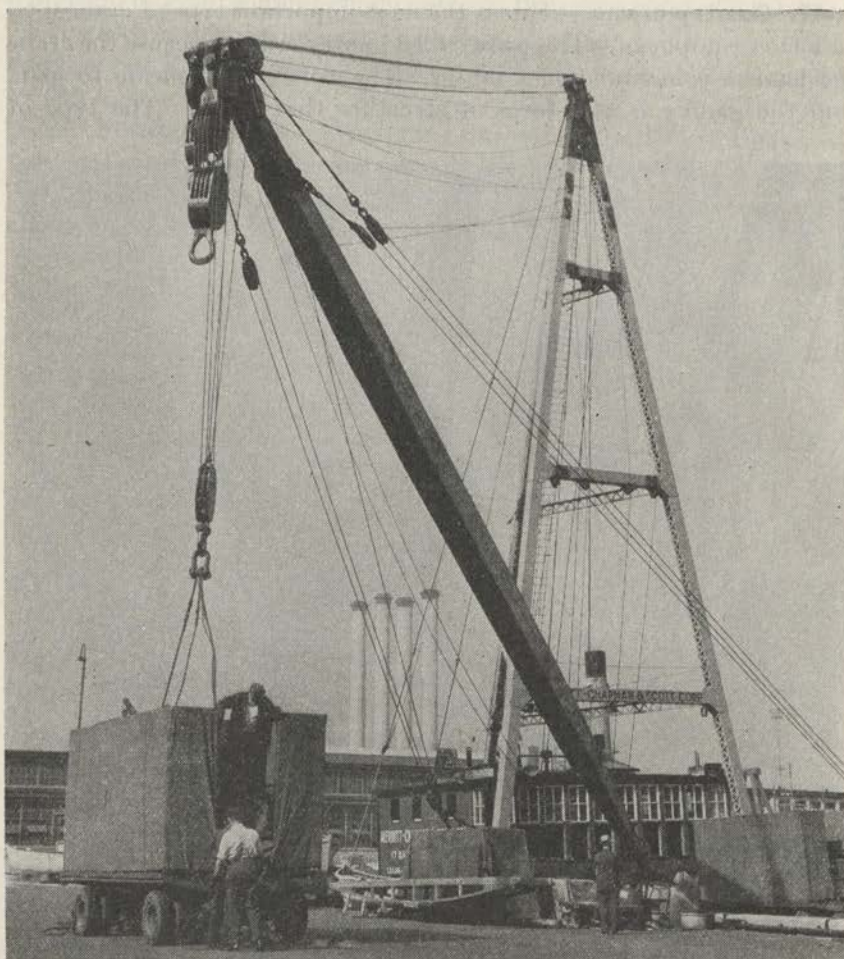
FIGURE 33.—Cables being attached to Army Air Force trailer for hoisting on barge.
