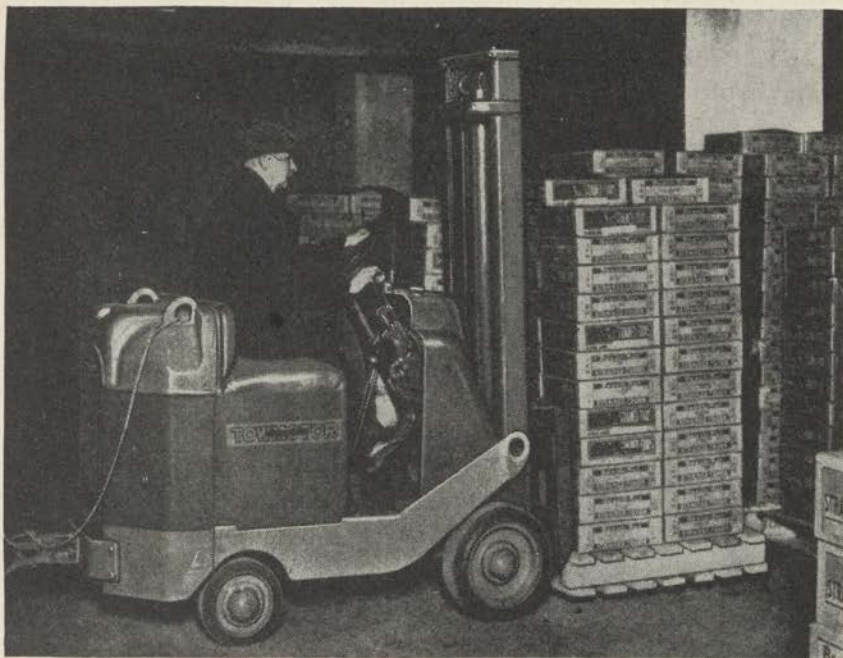
FIGURE 89.—Canned goods on "cooty" pallet.
