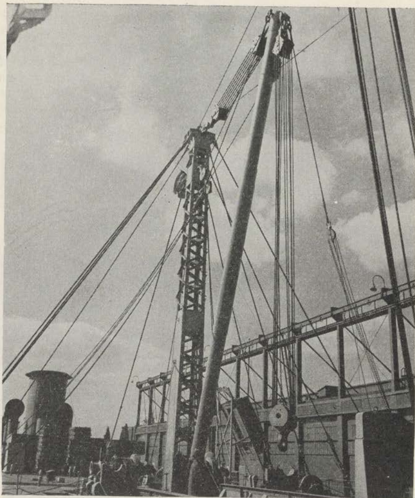
FIGURE 11.—An 80-ton boom, blocks, tackles, kingport, etc.
