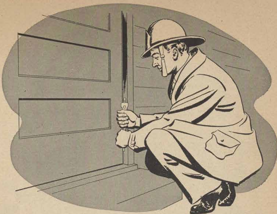
Figure 11. Hinge pins can be removed by tapping with ax or spanner wrench. This method saves damaging door or casing.
