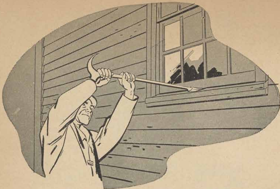
Figure 18. Method of opening check-rail window with window opener. Ax or spanner wrench may also be used.
