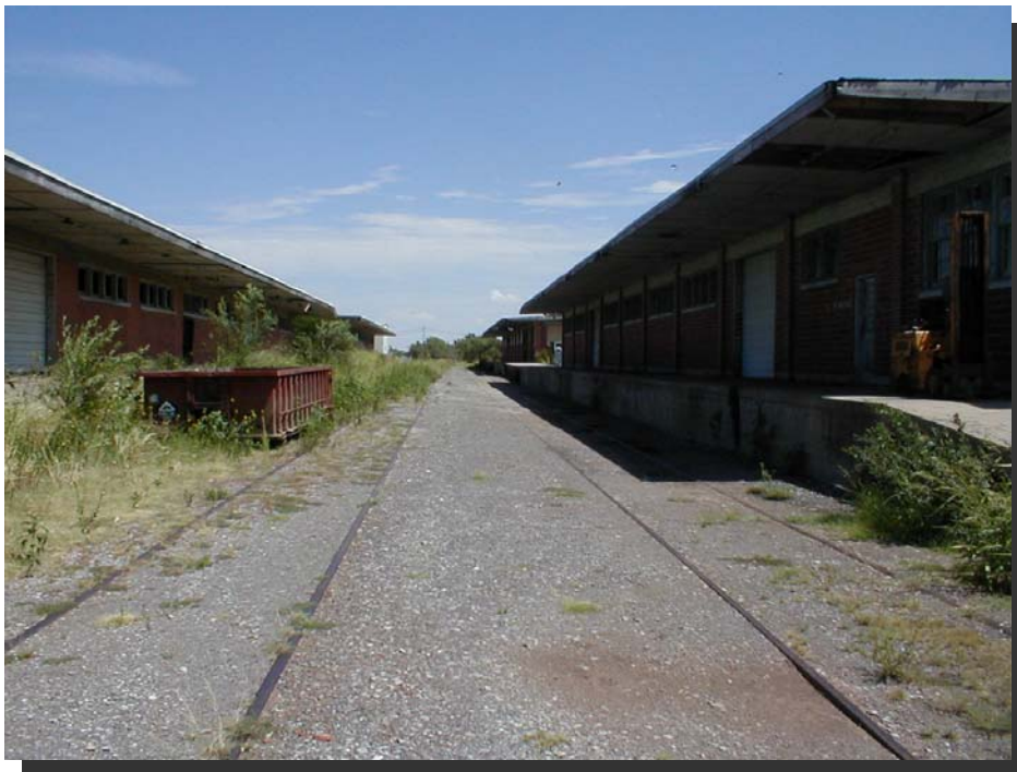
Exhibit 3-25. Rail Spur in Warehouse Area of CSIA
