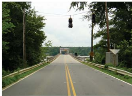
Shoulder widths less than current standards
