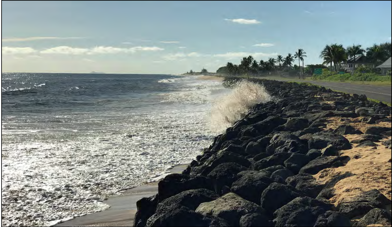
Figure 7.9. Wave striking a seawall protecting Kaumuali'i Highway on Kauai (Hawaii SH 50, 2018)
