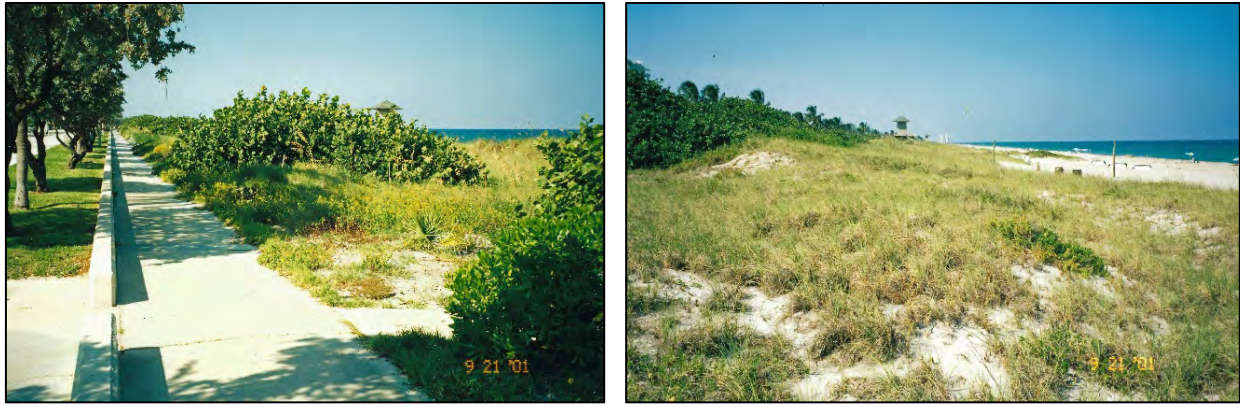
Figure 8.10. Beach nourishment project with constructed dune on top of old, failed revetment protecting Florida SH A1A (Delray Beach, 2001)
