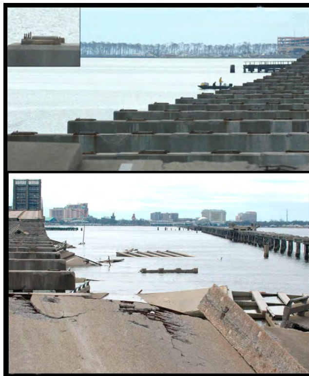
Figure 11.10. Details of damage to US 90 bridge over Biloxi Bay caused by Hurricane Katrina
