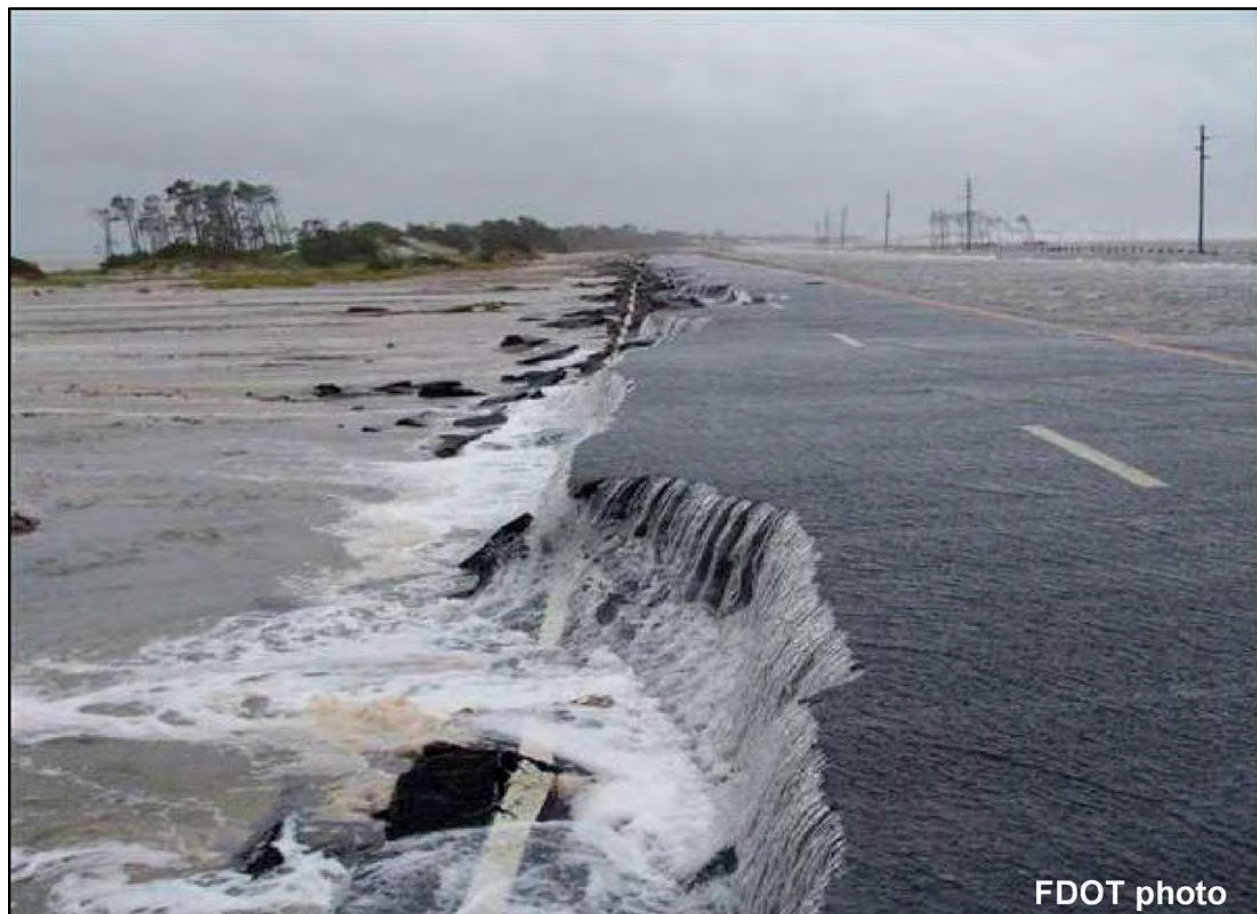
Figure 15.2. Example of the coastal weir-flow damage mechanism as it occurs (photograph provided by FDOT, circa 2005)
