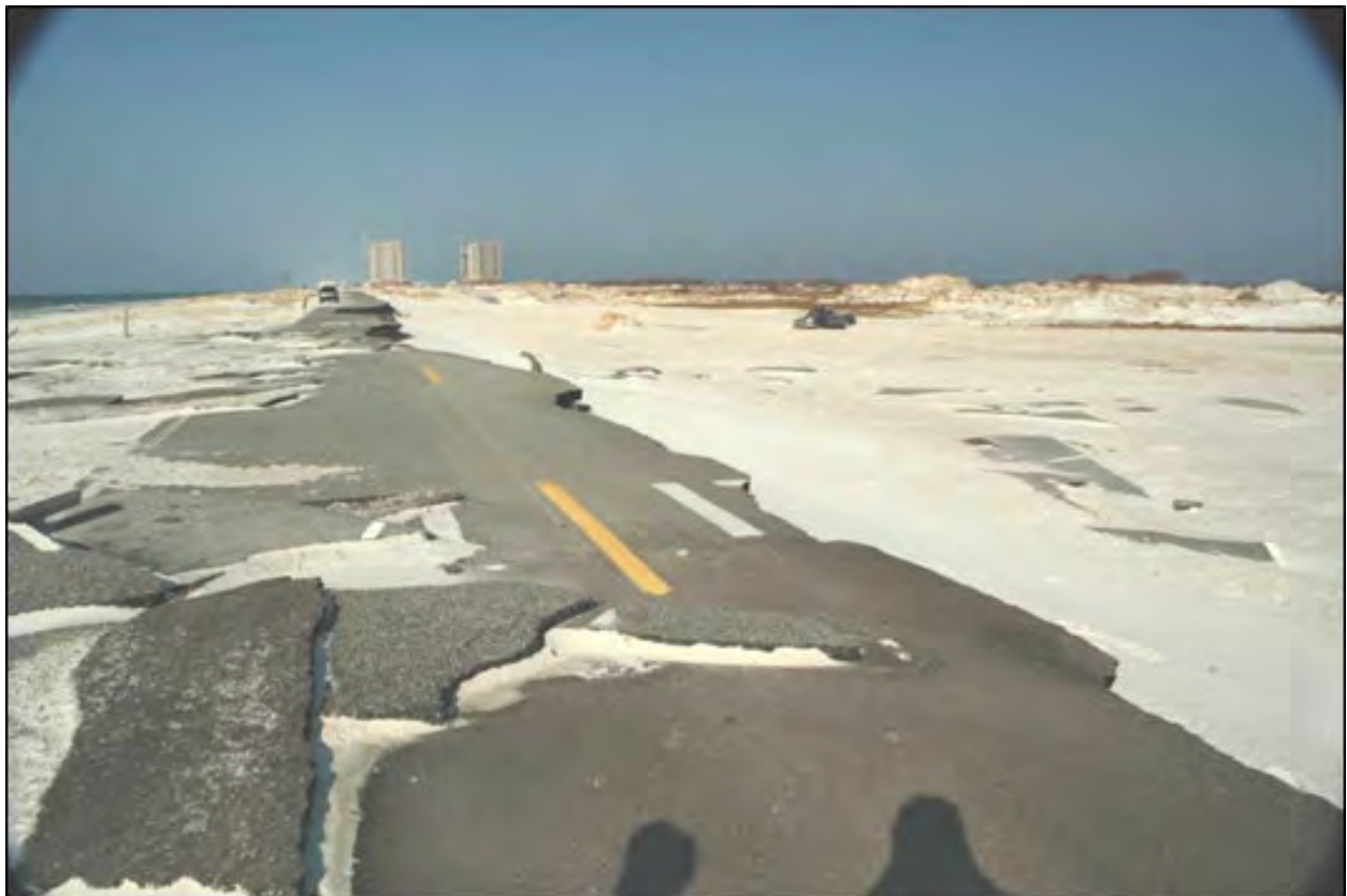
Figure 10.2. Example of pavement damaged by hurricane (photograph looking west on Florida SH 399, Gulf Islands National Seashore, 2005)
