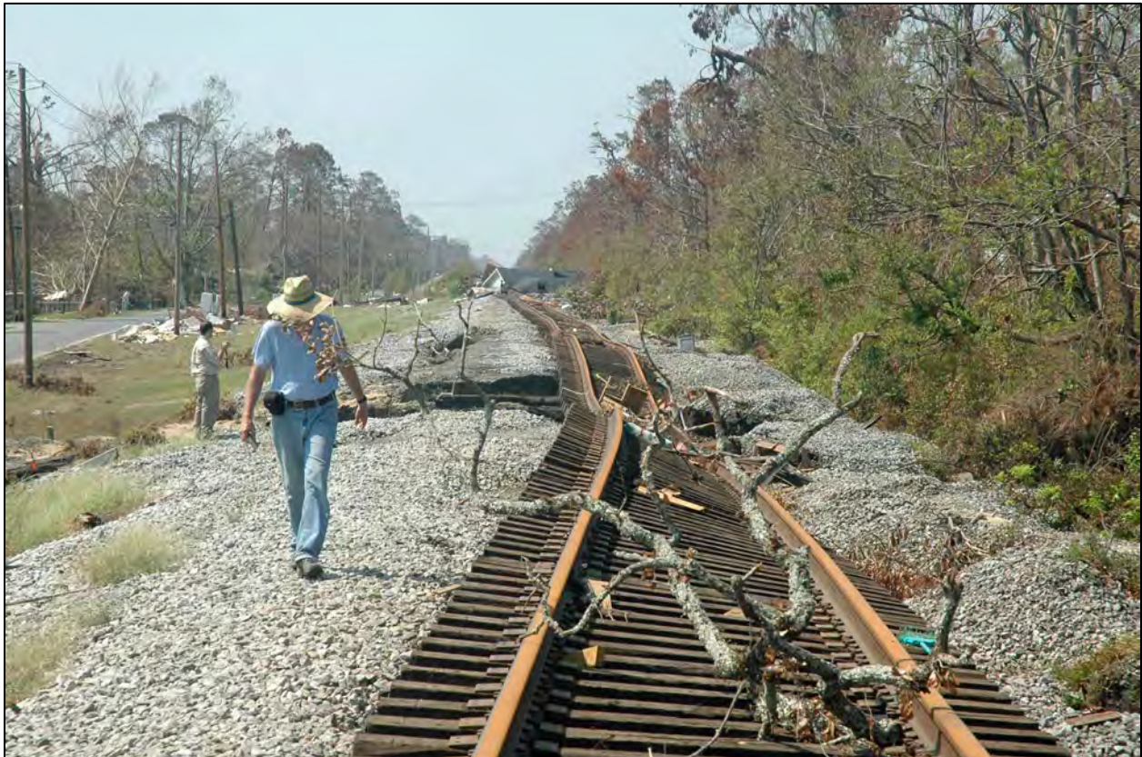
Figure 15.3. Railway embankment damage caused primarily by the coastal weir-flow damage mechanism during (Mississippi, 2005)
