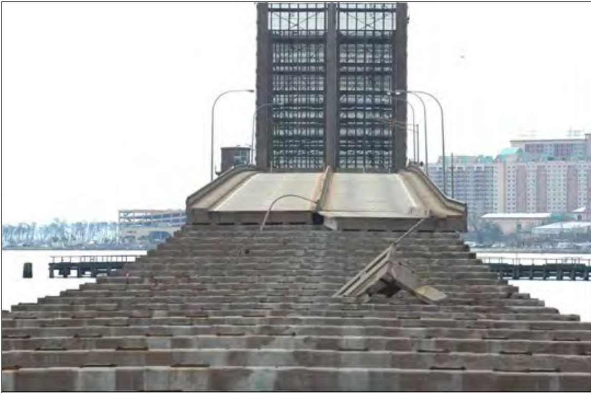
Figure 11.9. US 90 bridge over Biloxi Bay, Mississippi showing the spans below a critical elevation were removed by Hurricane Katrina (photograph looking southwest from Ocean Springs, February 19, 2016)
