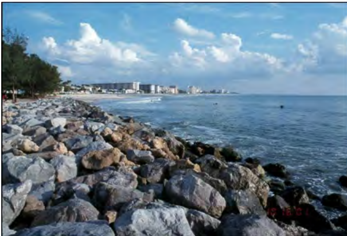
Figure 7.5. Seawall protecting a coastal highway (Venice, Florida, 2001)
