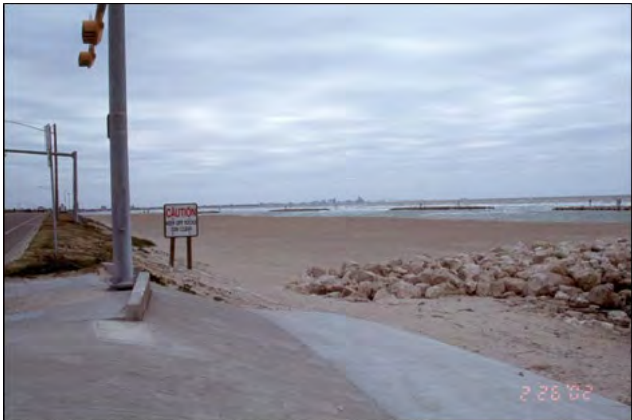
Figure 8.16. Offshore segmented breakwaters with groins and beach nourishment on Corpus Christi Bay (Ocean Drive, Corpus Christi, Texas)
