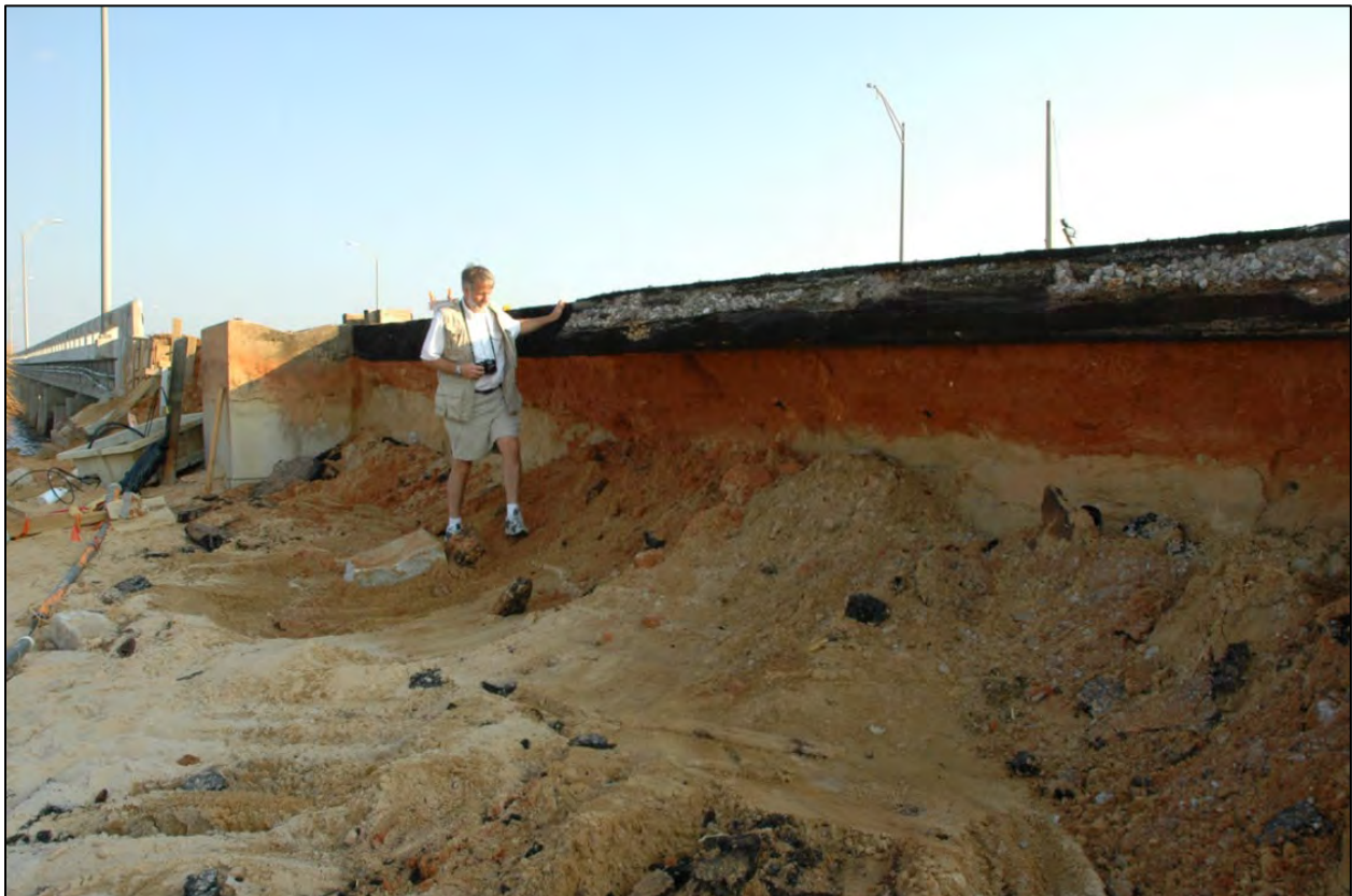
Figure 15.1. Partial embankment damage caused by waves on storm surge during Hurricane Ivan (Pensacola, Florida, 2004)
