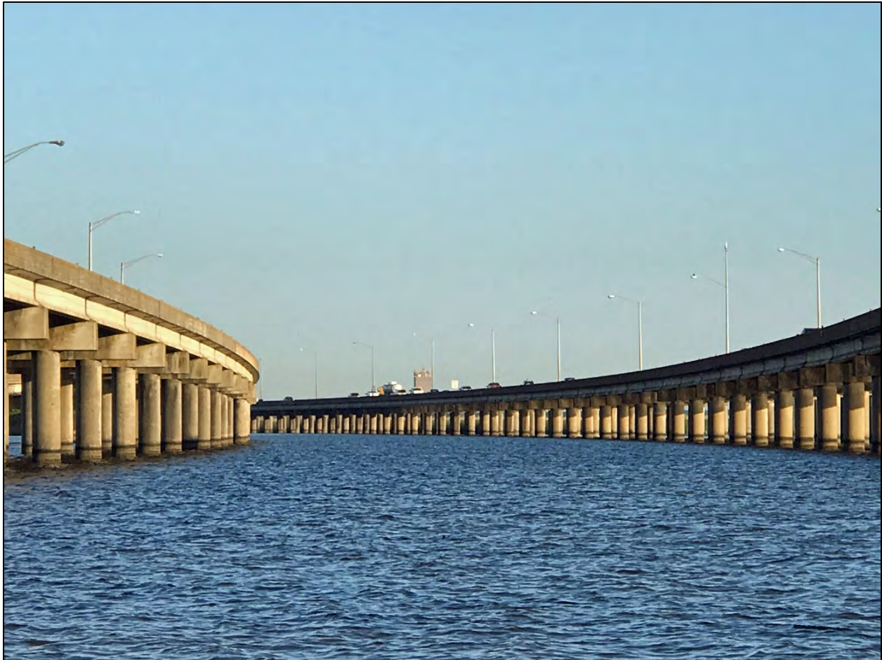
Figure 11.4. Interstate 10 bridge crossing Mobile Bay, Alabama
