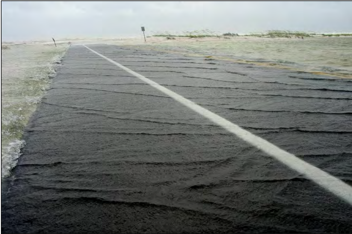
Figure 10.6. Weir-flow damage beginning (Fort Pickens Road, Gulf Islands National Seashore, Florida, July 2005; FHWA photograph)
