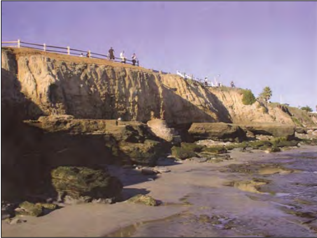
Figure 7.13. Concrete seawall designed to look like the natural rock formation built on an eroding sea cliff to protect a local road (East Cliff Drive, Santa Cruz, California, 2001)
