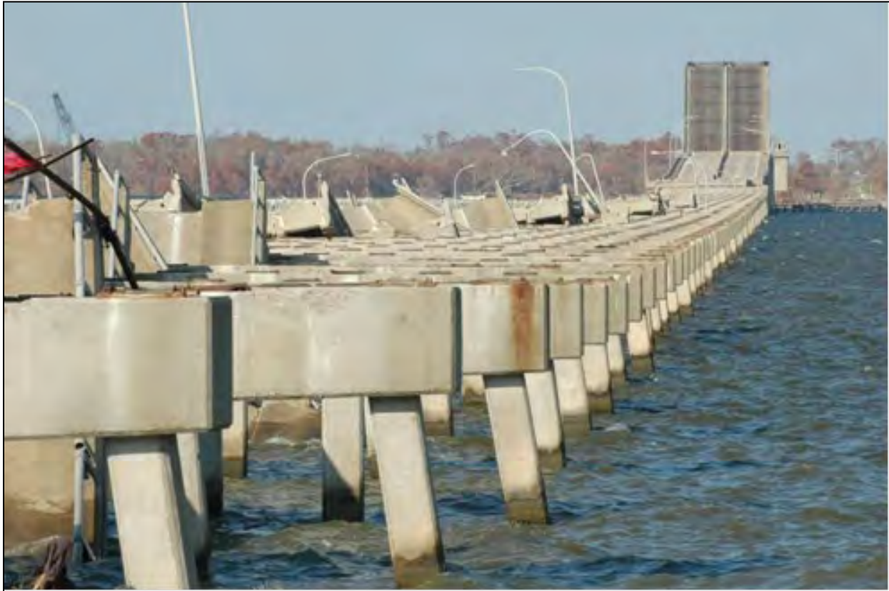
Figure 3.4. US Highway 90 bridge across Biloxi Bay, Mississippi, after Hurricane Katrina. (photograph looking northeast from Biloxi September 21, 2005)
