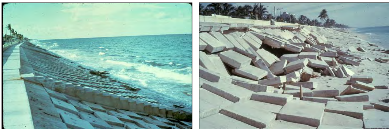
Figure 7.20. Example of rigid concrete-block revetment failure (Florida SH A1A, Delray Beach, circa 1972; University of Florida and USACE archive photos)
