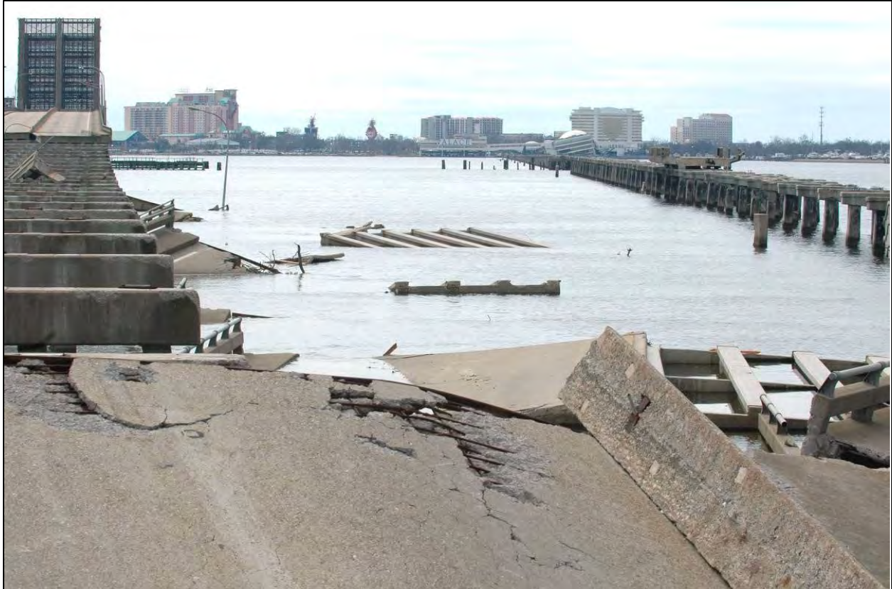
Figure 15.5. Two bridges destroyed by wave loads in Hurricane Katrina (Biloxi Bay, Mississippi)
