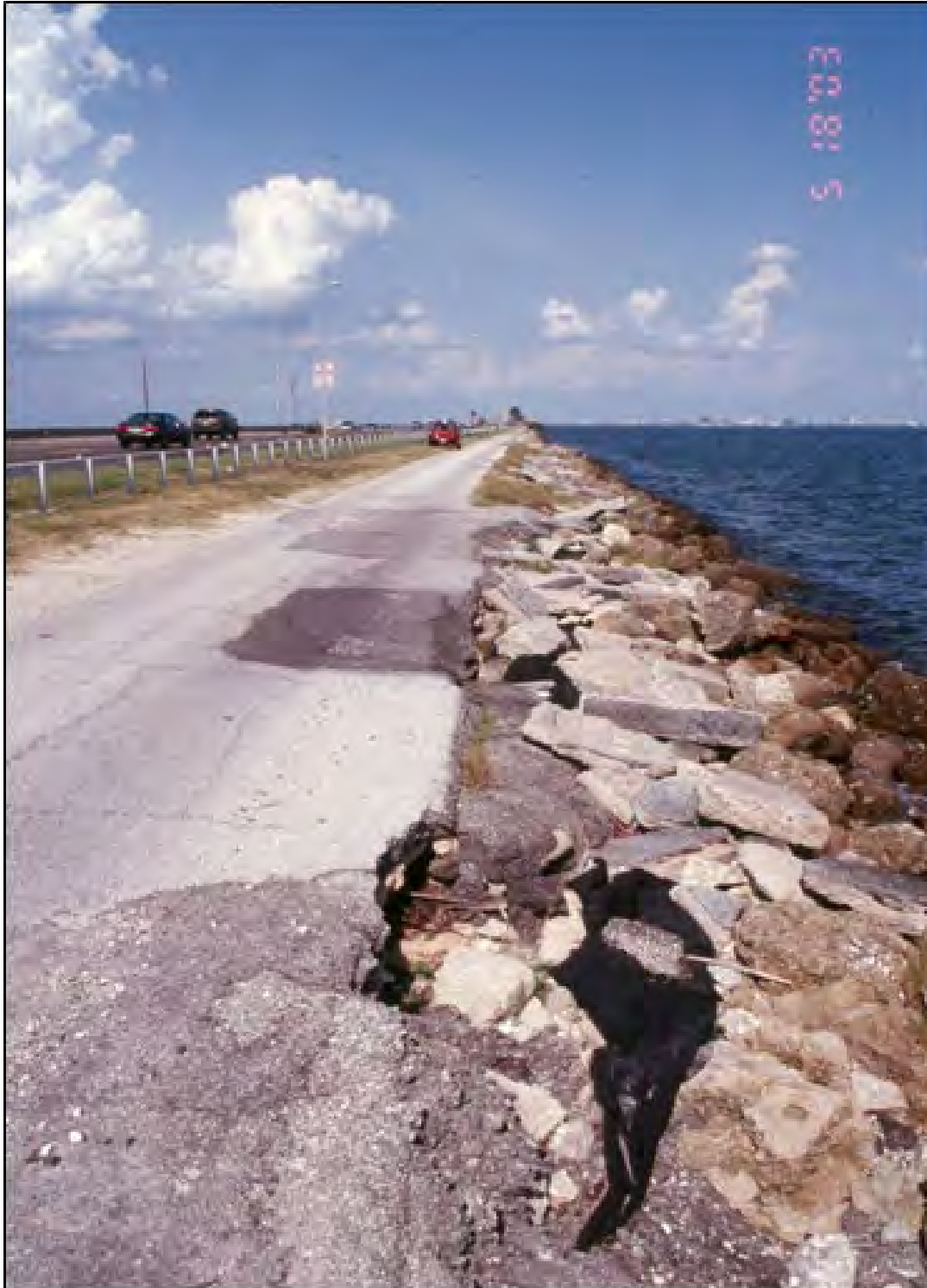
Figure 7.10. Revetment protecting a highway along a bay shoreline (Florida SH 60 crossing Tampa Bay, 2003)
