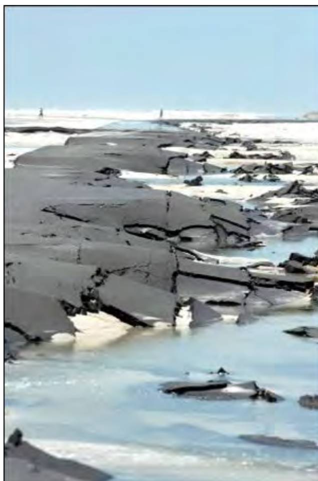
Figure 10.5. Pavement destroyed by the weir-flow mechanism (Fort Pickens Road, Gulf Islands National Seashore, near Pensacola, Florida)
