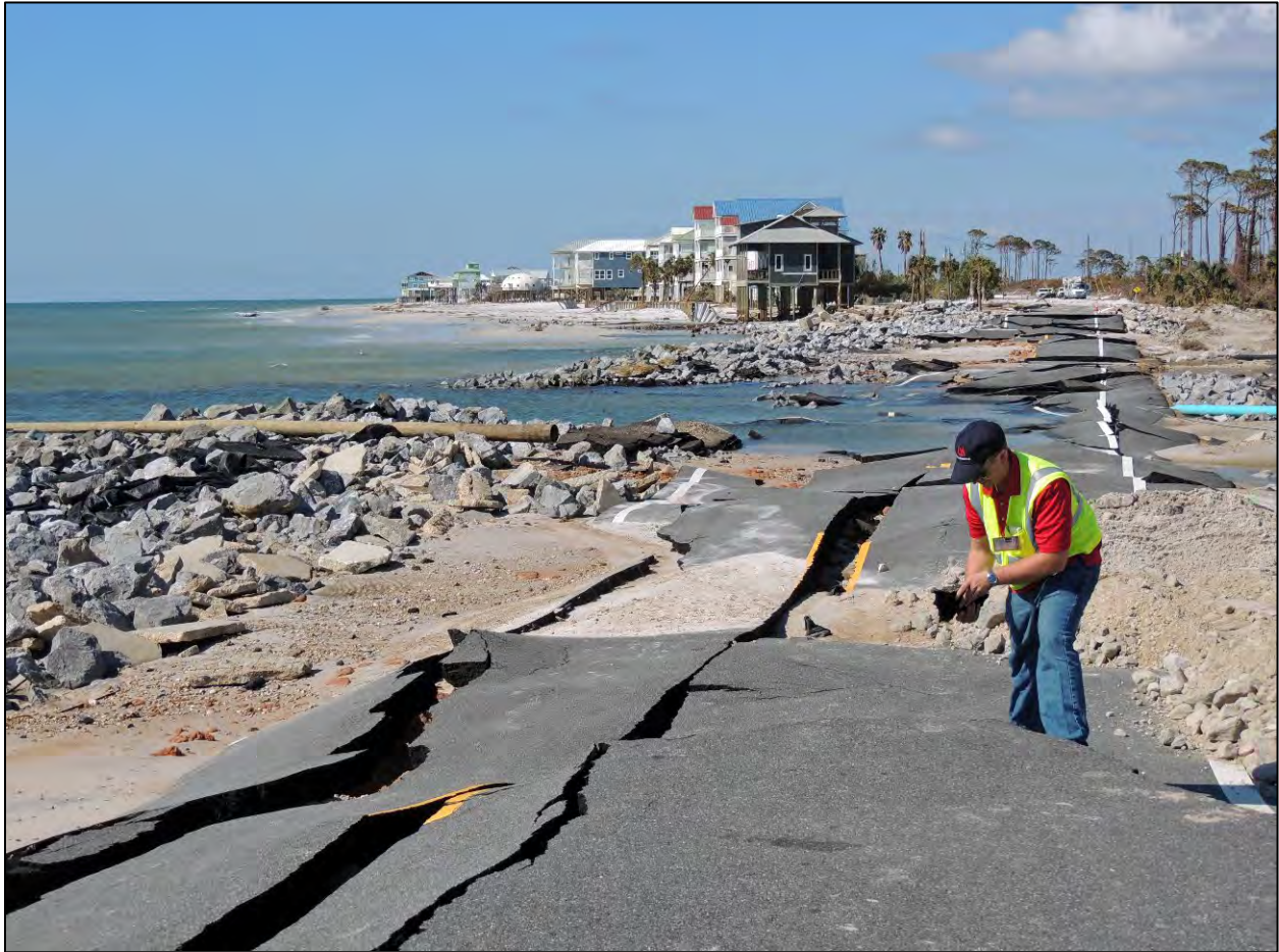
Figure 3.3. Damage caused by surge and waves in Hurricane Michael (October 14, 2018; permission to use photograph provided by John Cleary)
