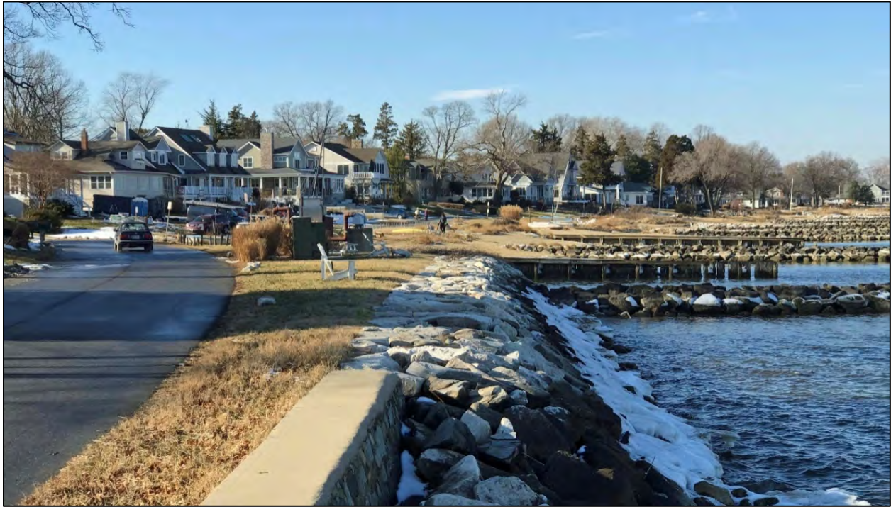
Figure 7.19. Example of a splash apron (center of photograph) at the top of a coastal rock revetment protecting a local road along a bluff on Chesapeake Bay (Shore Road, Anne Arundel County, Maryland, 2017)
