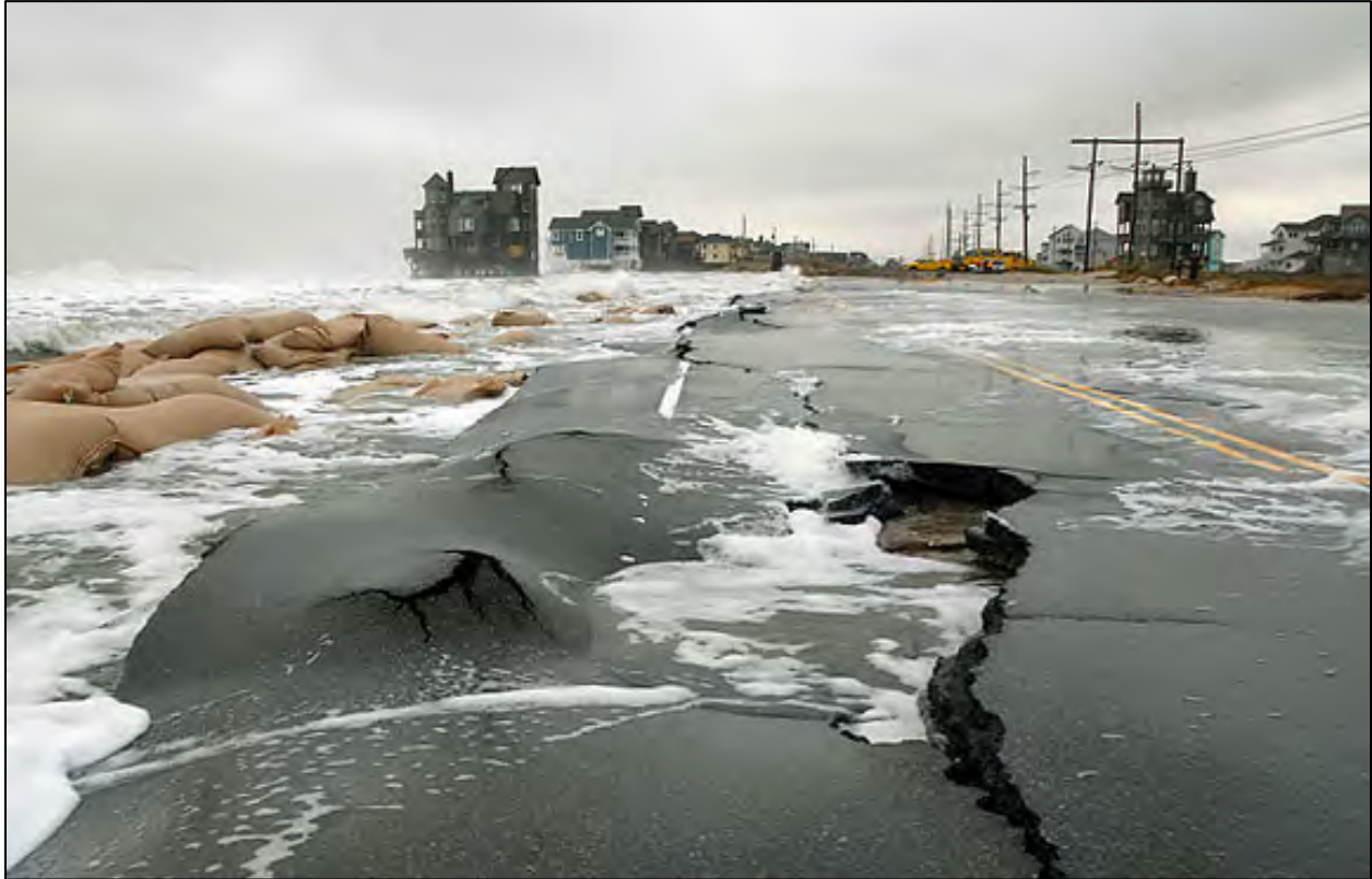
Figure 15.4. Pavement damage due to waves and surge in an extreme event (North Carolina SH 12, 2009; permission to use photograph provided by Dave Henderson)
