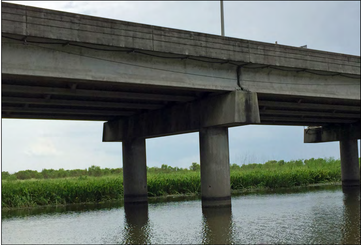
Figure 11.15. Example of concave seaward face of a coastal bridge (I-10 bridge over Mobile Bay, Alabama)
