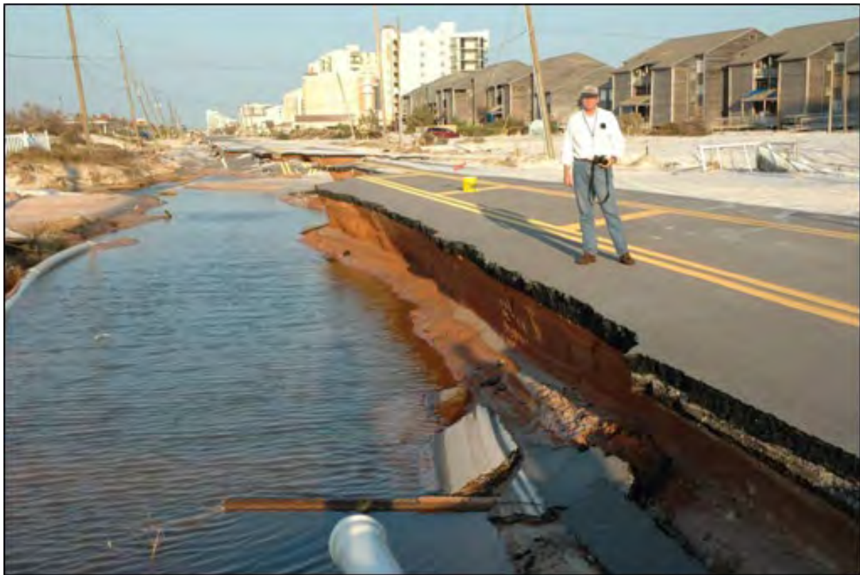
Figure 10.1. Example of pavement damage due to storm surge (Florida SH 292 on Perdido Key after Hurricane Ivan, September 2004).
