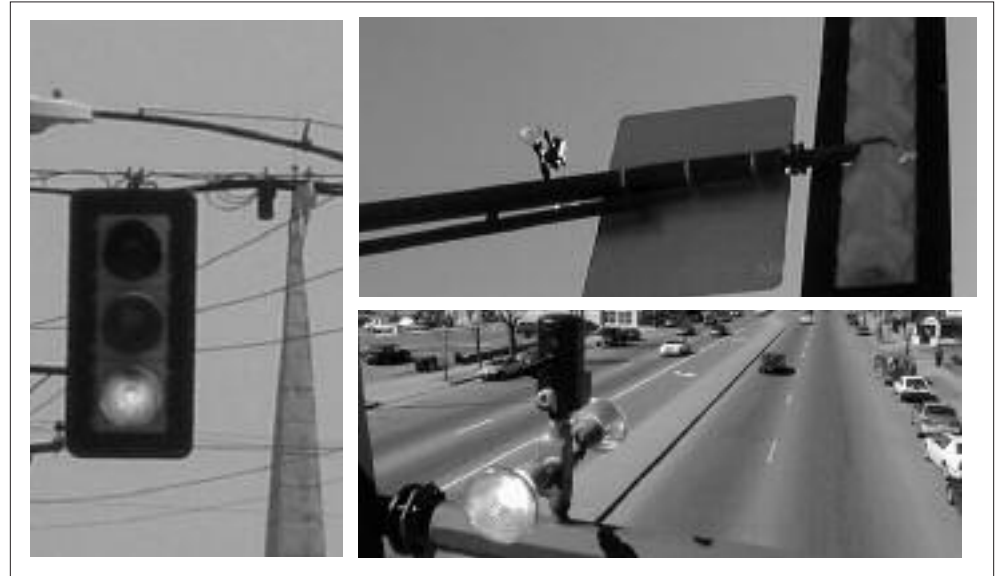
Figure 3 – Wire and Mast Arm Mounted Light-Based Detectors
