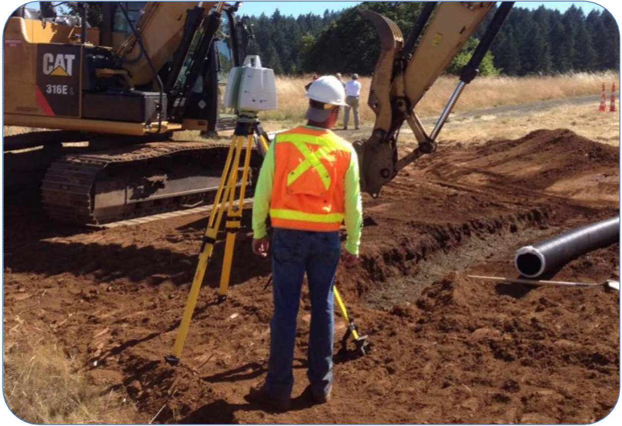
Figure 44. Photo. Static LiDAR being used to collect as-built data.
