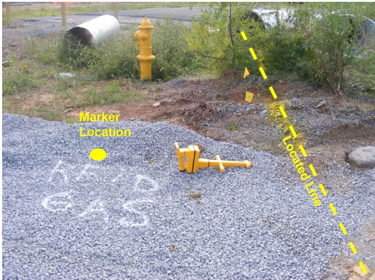
Figure 70. Photo. Discrepancy between one-call locate and RFID marker location. (11)
