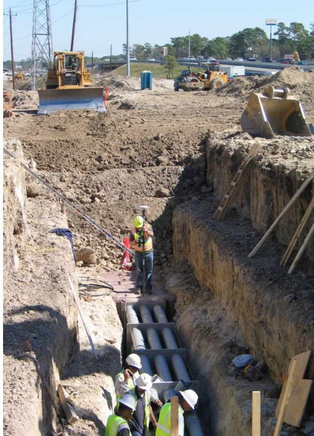
Figure 29. Photo. Collection of coordinate data for electric transmission duct bank.
