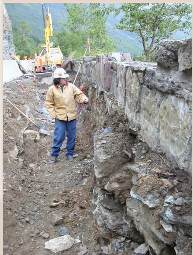
FHWA Resident Engineer Margaret Moen, who worked on the project until early 2006, inspects a construction site where a new and hidden concrete retaining wall was constructed inside the original wall, allowing the historic wall to maintain its original appearance without having to support its former structural load.
