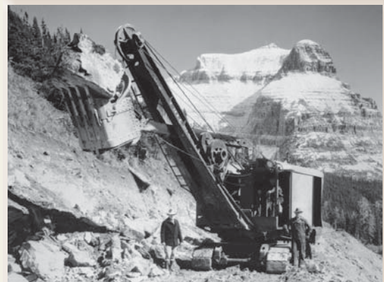
A crew uses a power shovel east of Logan Pass in 1932. Going-to-the-Sun Mountain, for which the road is named, is seen in the background.
