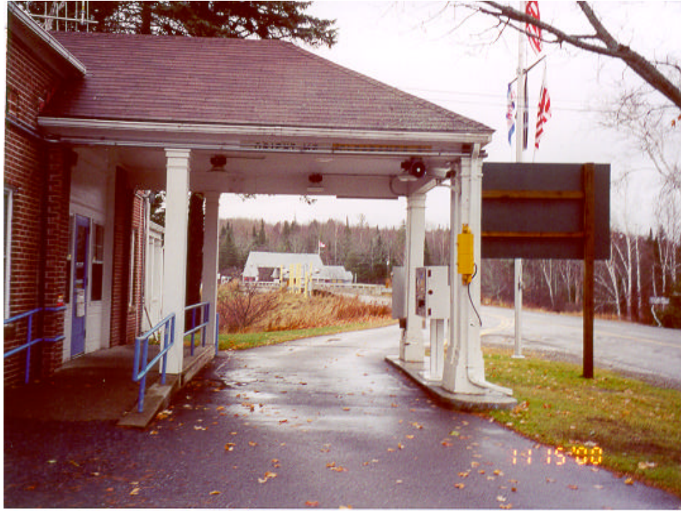
Figure 4: Border Crossing at Orient, Maine
