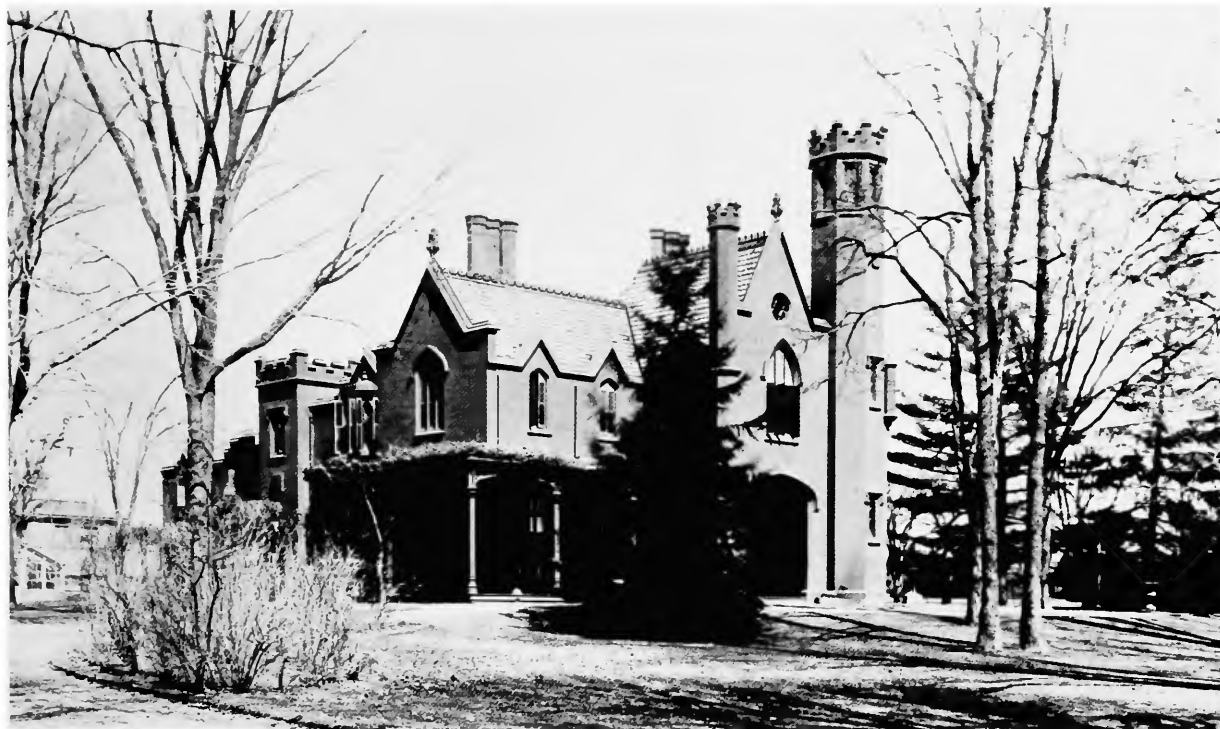
Figure 4. The brick walls of the house were stuccoed and scored to simulate stonework. The Bridgeport Republican Standard of August 1, 1848, reported that another house nearby was being stuccoed; this was done under the direction of a Mr. Gill from New Haven "... who has a high reputation in the stucco line. The finish and durability of his work have tended very much to change the opinion of the public in reference to the value of this material for building purposes. It is now preferred by competent judges, for the most expensive edifices." (Smithsonian negative 68114.)
