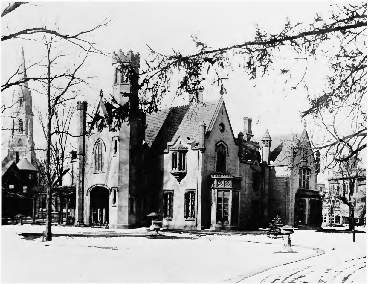
Figure 8. Compared with Davis's plan for an addition to the Harral residence, the library built in 1866—seen in this photograph as the projecting bay at the back of the house—was undistinguished. Fortunately, however, it was compatible with the established architectural style. (Smithsonian negative 68115.)
