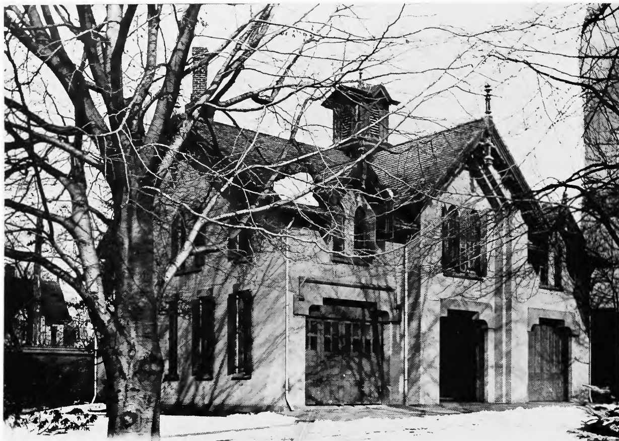
Figure 9. Davis's coach house and stable was replaced soon after Nathaniel Wheeler acquired "Walnut Wood." The Bridgeport Evening Standard of October 24, 1866 commented "We notice that Mr. N. Wheeler, has commenced to excavate for a new barn, for the Harral Place on Golden Hill. The barn is to be a splendid one, and was designed by those excellent Architects, Messrs. Lambert & Bunnell. The building is to be of pressed brick, with 50 feet front. The main part will be 54 feet on the side, with a wing 22 by 33 feet. The wing is to have 8 nice stalls. The carriage room will be 38 by 34 feet, and the harness room 10 by 14. The loft extends over the whole building." (Smithsonian negative 68112.)
