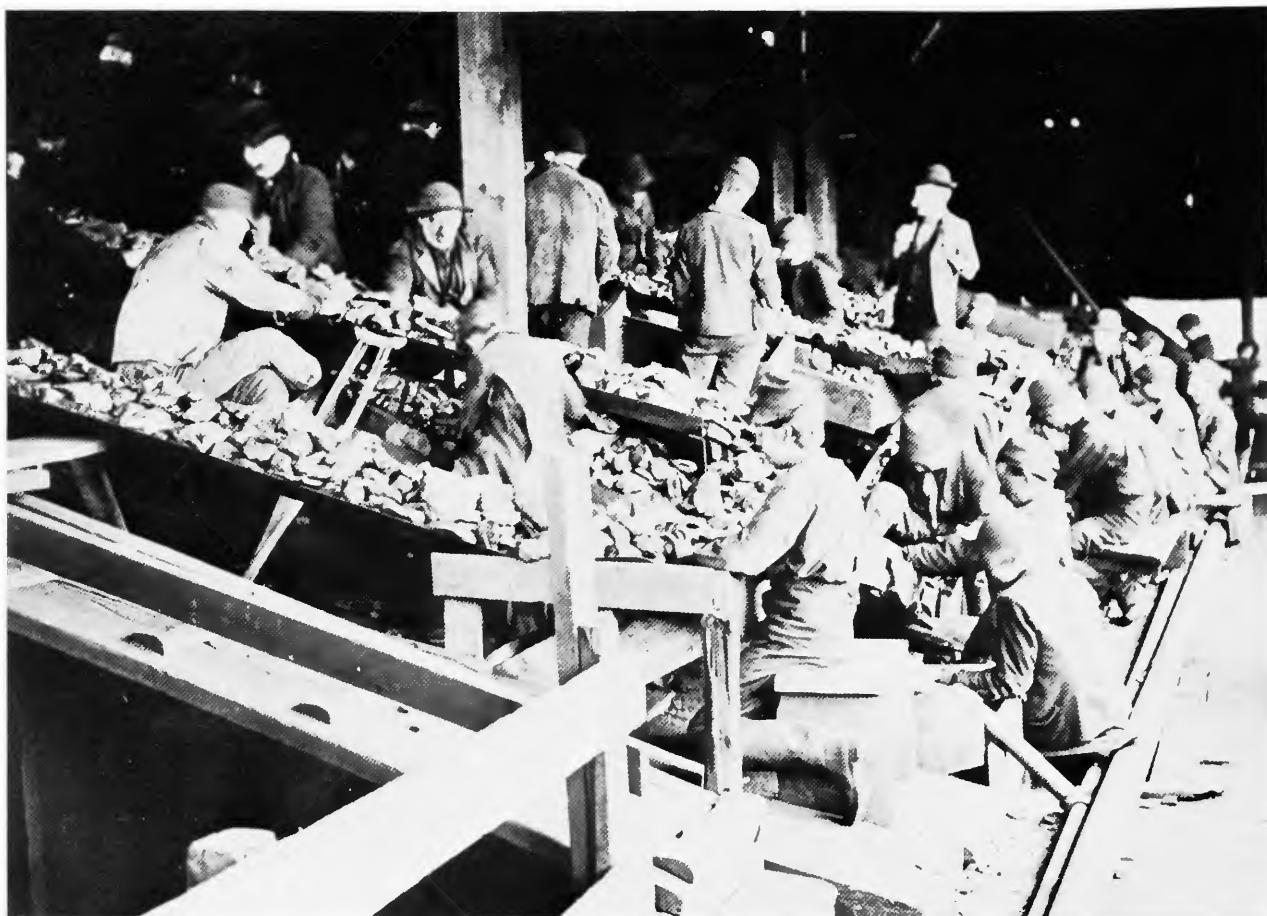
FIGURE 29.—Examples of breaker-boy operations. (Photograph courtesy of the Girard Estate.)
