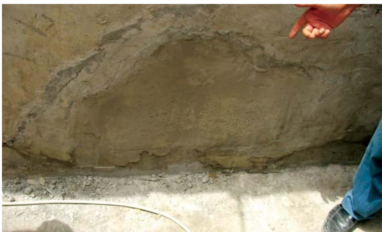
Unacceptable cement pour at a Falluja Waste Water Treatment System pump station.
