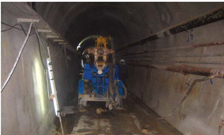
Grouting equipment in the tunnel under the Mosul Dam during SIGIR inspection.
