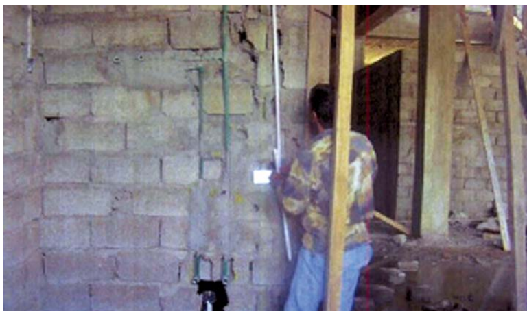
Example of poor block laying at primary healthcare center in Kirkuk. (USACE photo)
