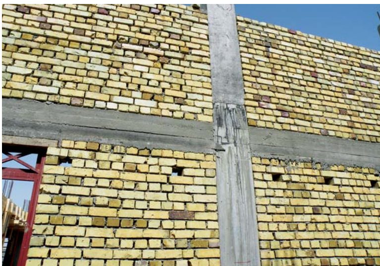
Basrah Modern Slaughterhouse under construction, showing upper-level concrete intermediate (cross) beams improperly supported by brick façade.
