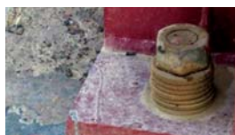
Poor installation technique (use of seven washers).
