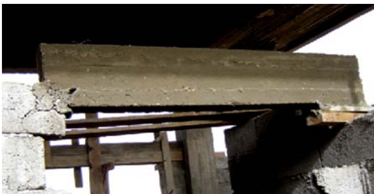
Improper support for a load-bearing lintel at a primary healthcare center during construction. (USACE photo)
