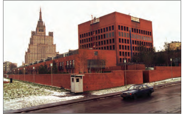
Figure 15: The New Office Building at the U.S. Embassy in Moscow. Due to the bugging system discovered in the structure of the red brick building, the United States expelled the Soviet workers, tore down the upper floors (to the base of the fifth floor), inserted shielding to prevent any new bugs, and rebuilt the upper floors. Soviet workers arranged darker colored bricks so that one could read “СССР” (Russian for USSR) in the façade of the U.S. Embassy. Source: © Associated Press.
