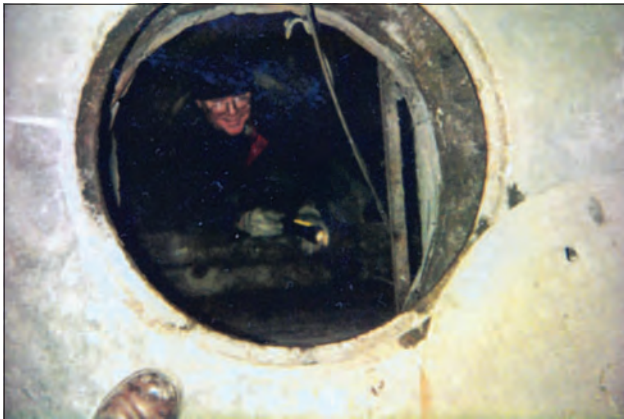
Figure 6: Winter 1994: A DS Security Engineering Officer works to install alarms in the utility tunnels beneath a U.S. embassy overseas. The alarm system was a precautionary countermeasure aimed at alerting embassy security personnel if intruders entered the tunnels. Running beneath public streets, such tunnels sometimes were used in espionage efforts by foreign intelligence operatives. Source: Private collection.
