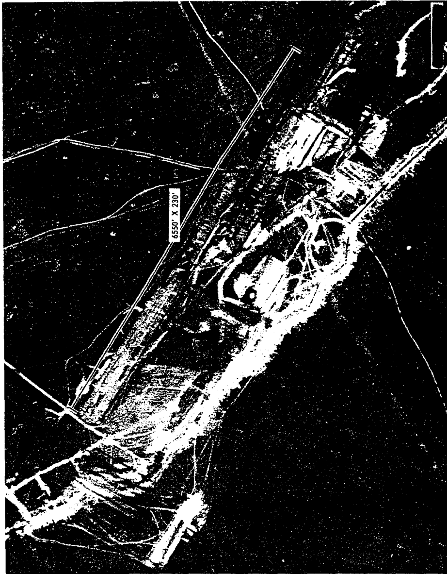
AIRFIELD UNDER CONSTRUCTION, CHOYBALSAN, MONGOLIA (AIRFIELD BONUS)
